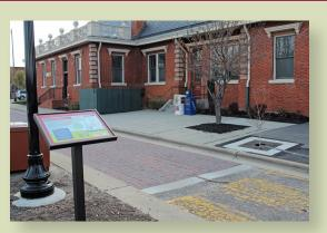
permeable pavement and a stormwater bio-retention system to help treat stormwater runoff. This system will capture and immobilize stormwater pollutants to treat runoff in the immediate area. Pollutants such as nitrogen, phosphorous, and oils will be filtered out of the runoff before being discharged into the City's storm drainage system. For more information regarding the City's stormwater division, please visit
