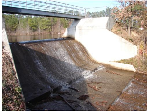
The spillway controls the flow of water out of Glenville Lake downstream into the Little Cross Creek
