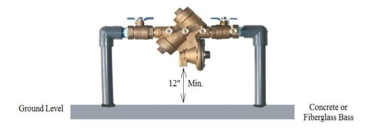
An above ground enclosure that covers the backflow preventer is required. This is to protect the backflow preventer from freezing.
