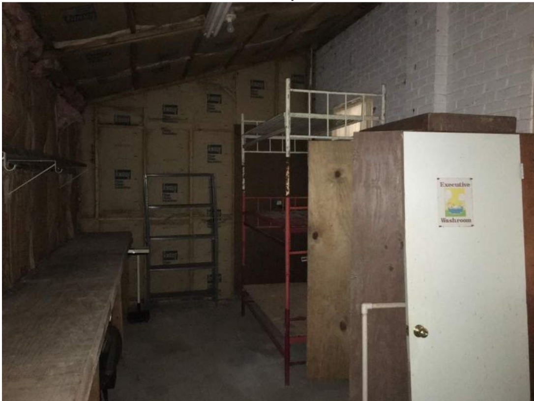
Photo 46: Storage Shed, Viewed from Doorway to East Wall
