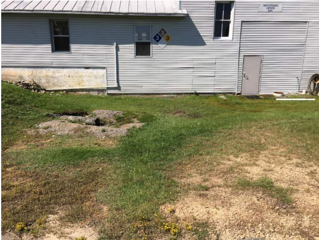
Photo 9: Catch Basin 1 Area, Viewed from East
