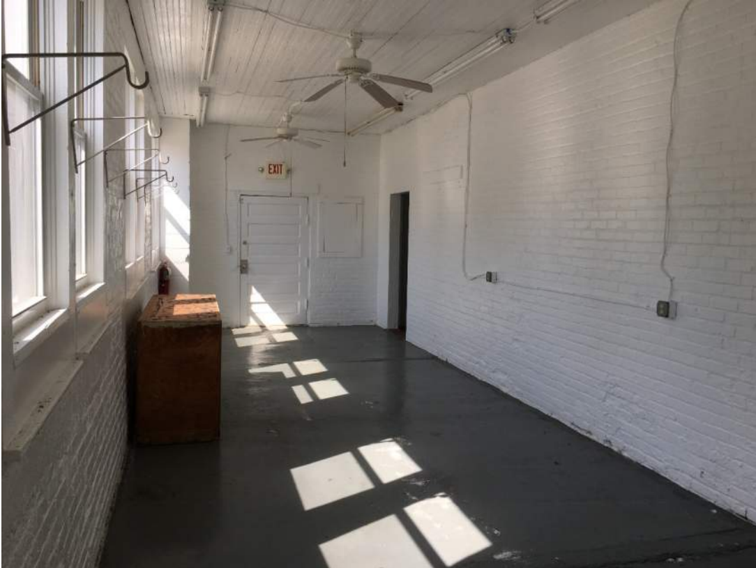
Photo 39: Hallway #2, Viewed from East Wall to West Wall
