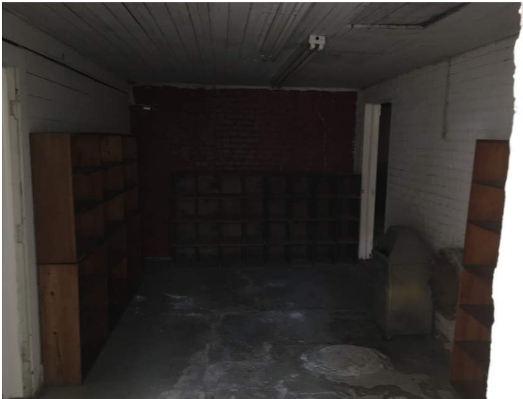
Photo 44: Storage #2, Viewed from South Wall to North Wall
