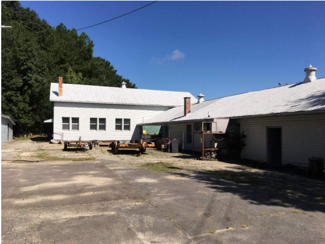
Photo 5: Former WTP Building Western Exterior, Viewed from Southwest
