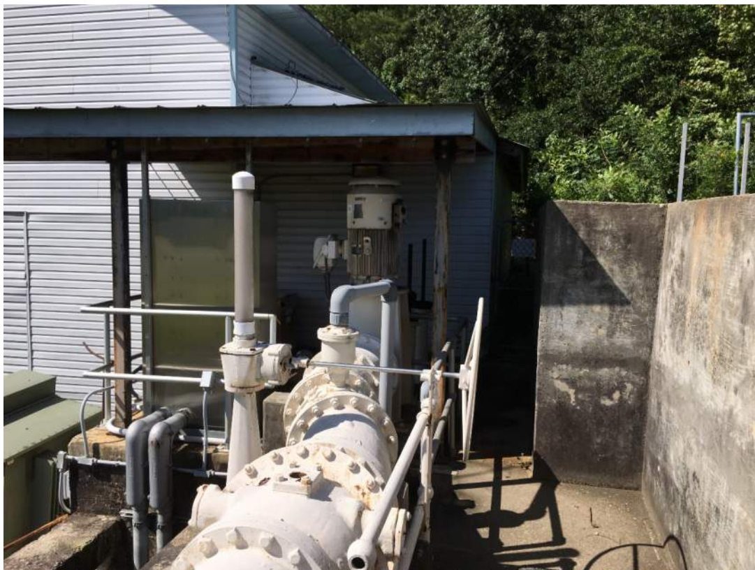
Photo 12: Raised Wet Well Pumping Platform, Viewed from East
