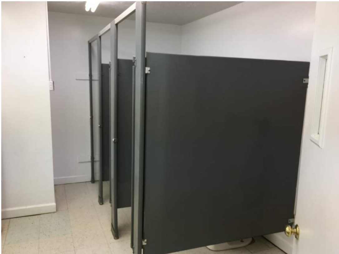
Photo 18: Bathroom #1 Toilet Stalls
