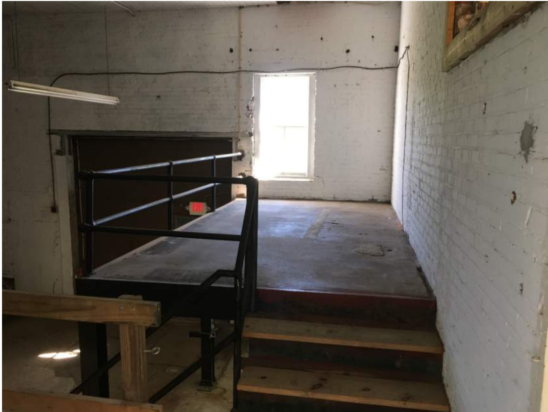
Photo 33: Upper Level North Room, Viewed from Southwest Corner to East Wall
