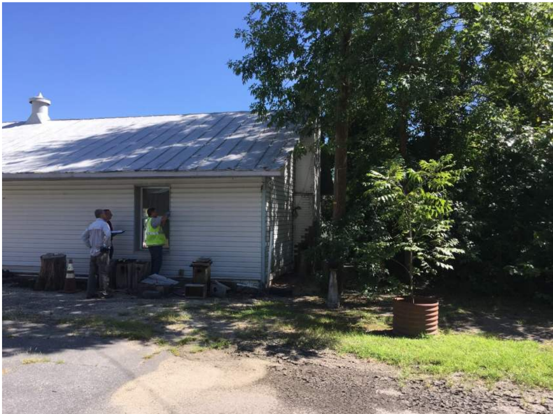
Photo 4: Former WTP Building Southwestern Exterior, Viewed from Southwest
