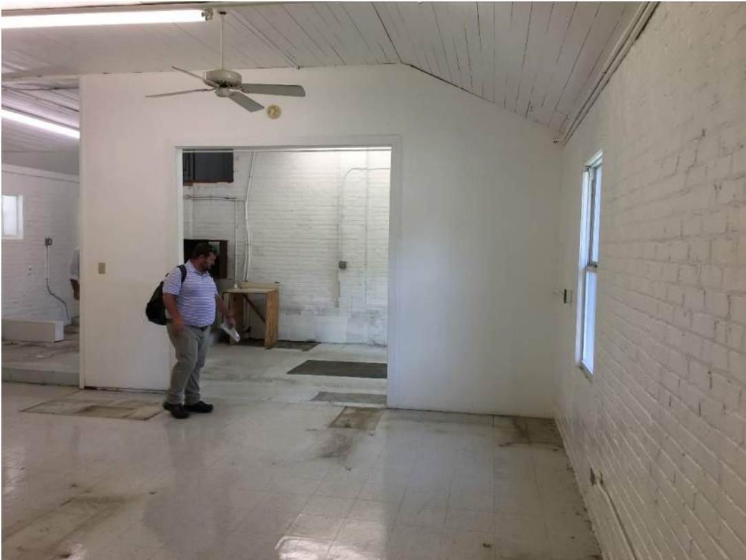
Photo 30: Middle Room, Viewed from Southeast Corner to North Wall
