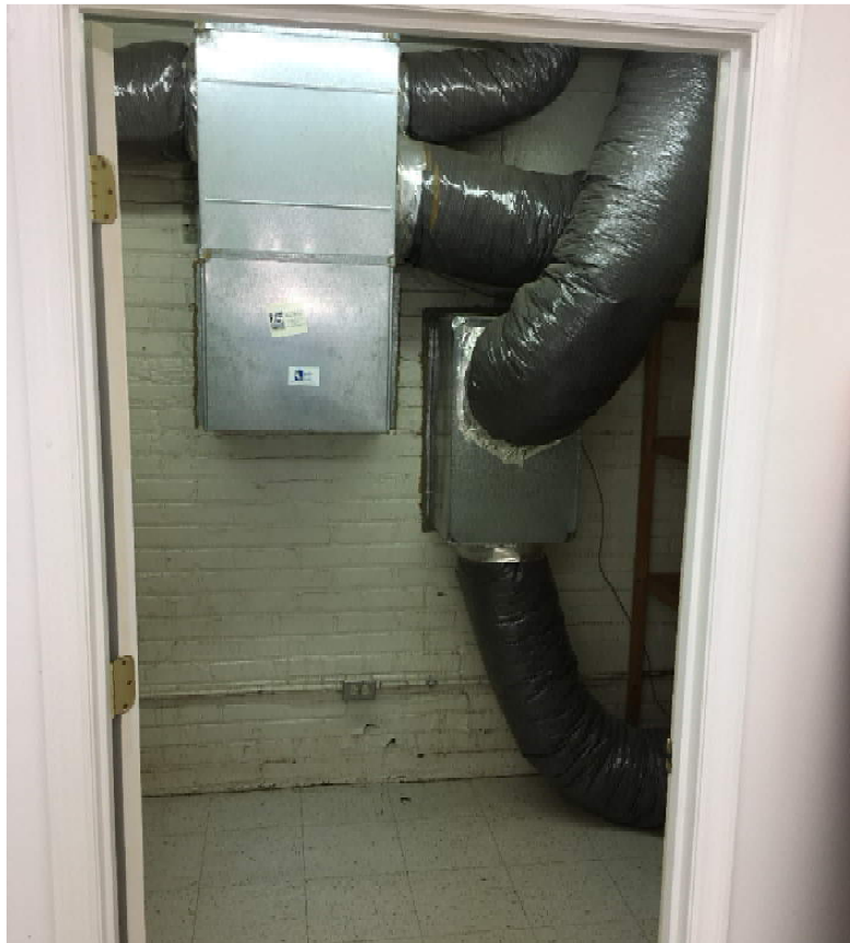
Photo 26: Storage #1, Viewed from Doorway
