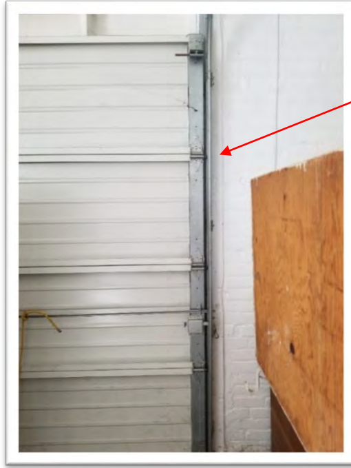
Photograph #0013 White Lead-Based Paint associated with wood garage door casing in the Kitchen
