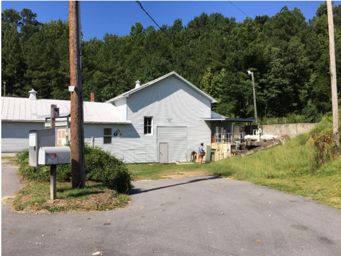
Photo 3: Former WTP Building Northeastern Exterior, Viewed from East
