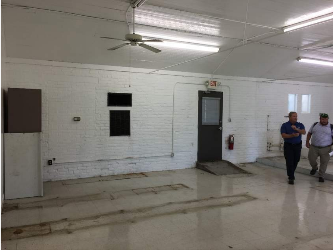
Photo 29: Middle Room, Viewed from Southeast Corner to West Wall
