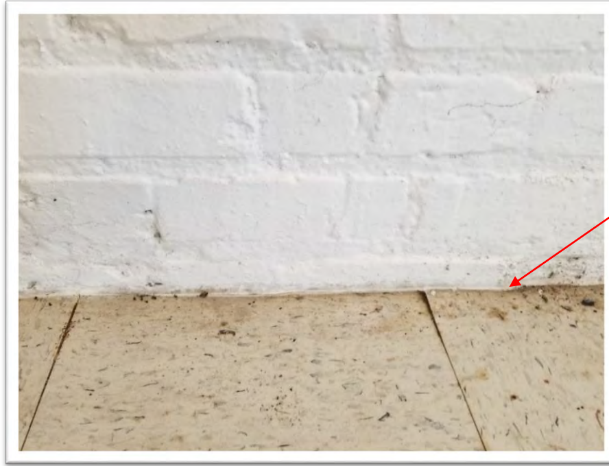
Photograph #0003 Base Caulking between floor and wall in the South Room
