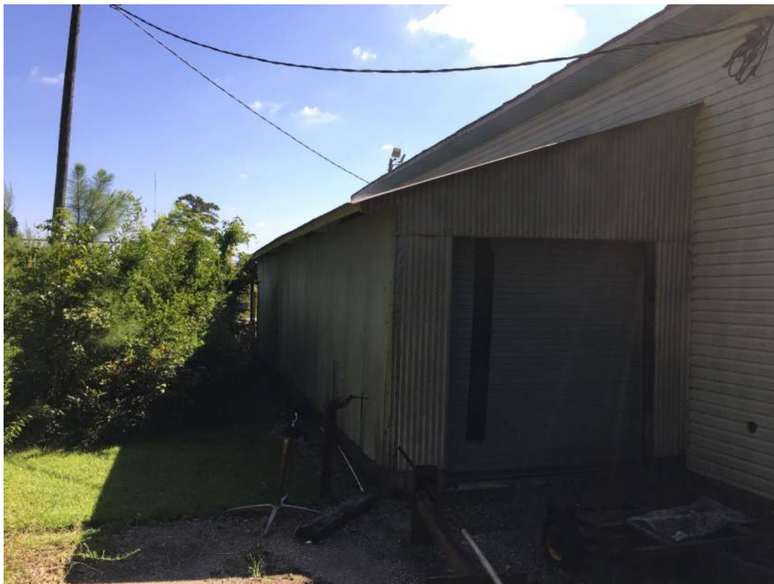
Photo 7: Former WTP Building Northern Exterior, Viewed from Northwest
