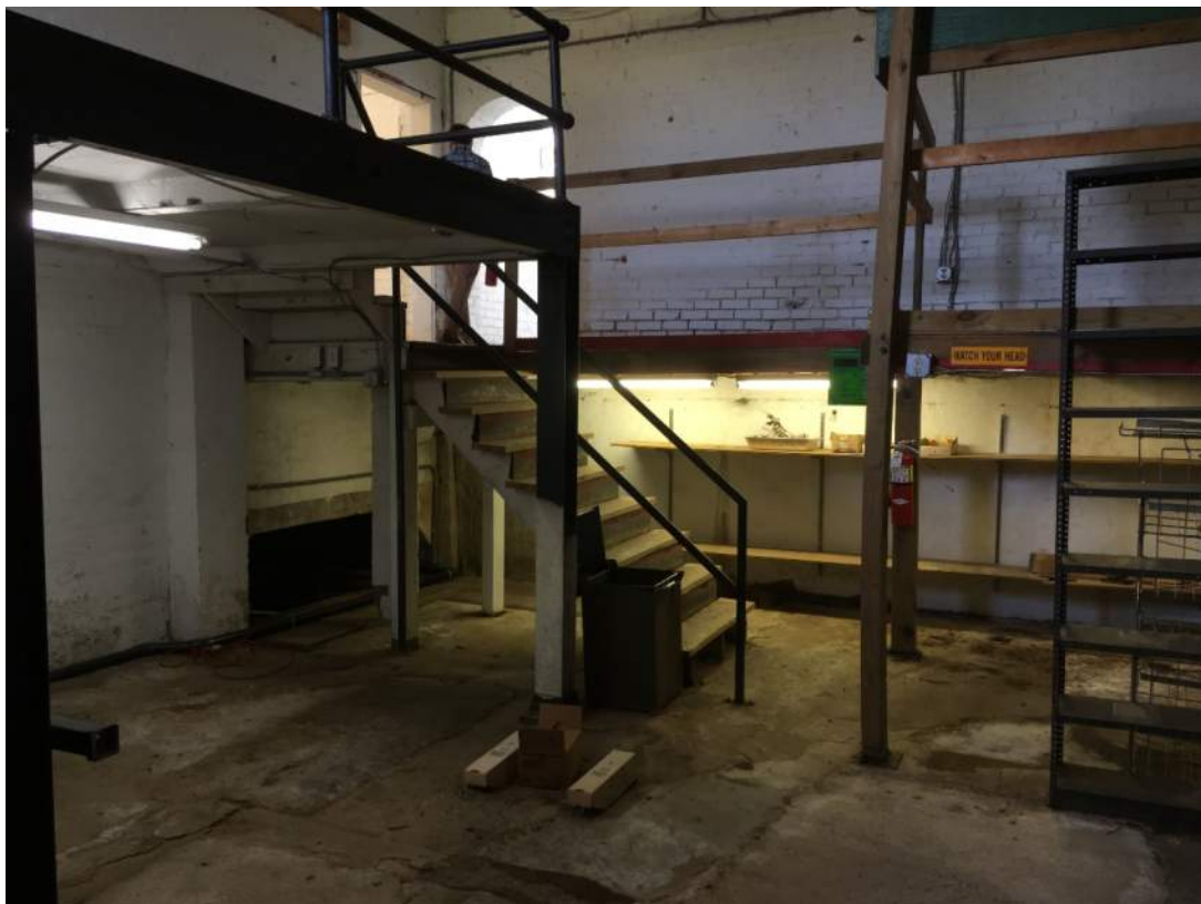
Photo 37: Lower Level North Room, Viewed from East Wall to Southwest Corner towards Pipe Gallery
