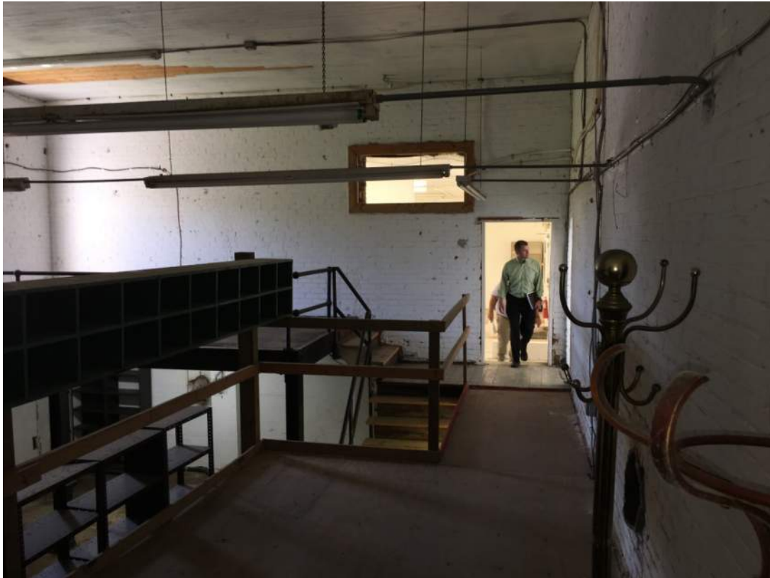
Photo 31: Upper Level North Room, Viewed from Northwest Corner to South Wall
