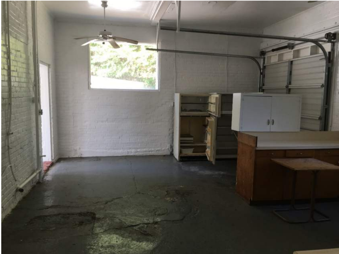
Photo 41: Kitchen, Viewed from East Wall to West Wall
