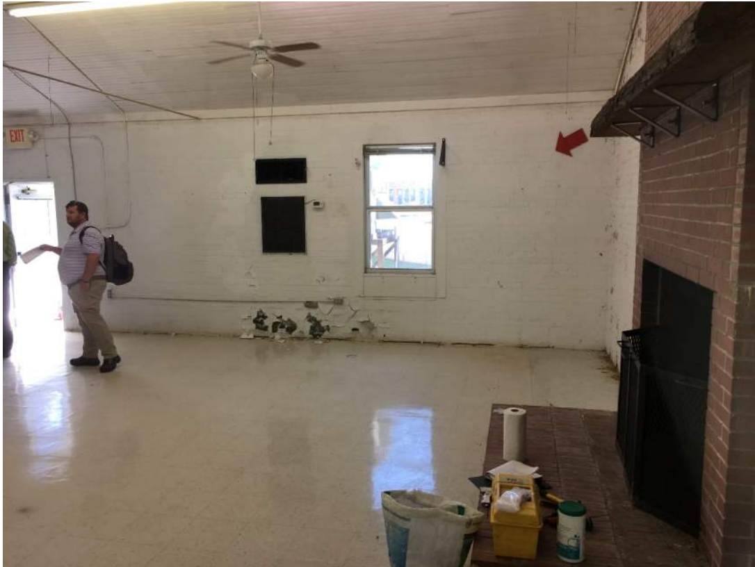
Photo 15: South Room, Viewed from Southwest Corner to East Wall
