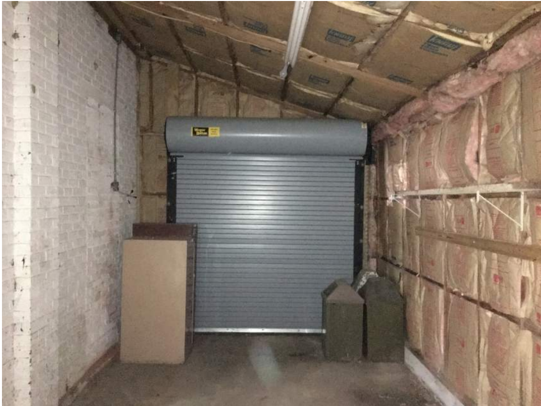
Photo 45: Storage Shed, Viewed from Doorway to West Wall
