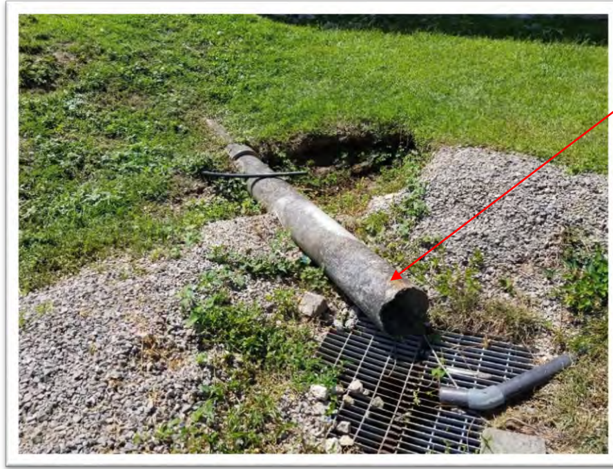
Photograph #0003 East Wing Exterior– Semi-buried Cement Fiber Pipe
