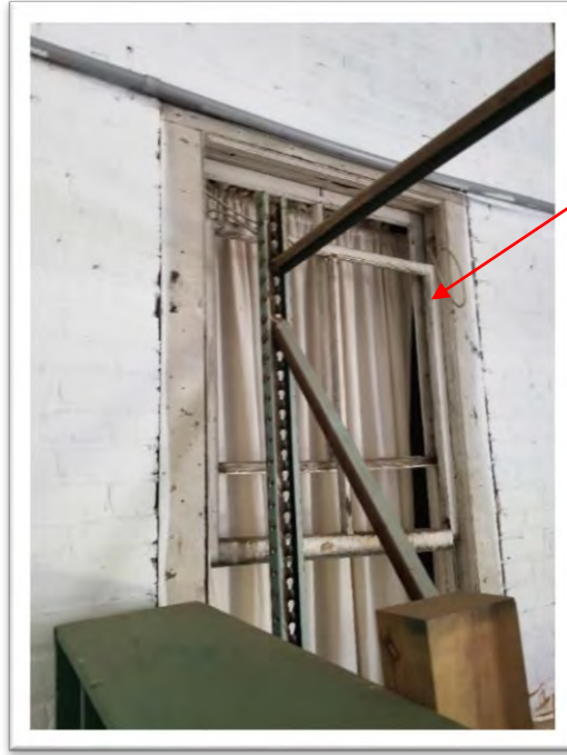
Photograph #0009 Off-White Lead-Based Paint associated with wood window casing & sash in North Room
