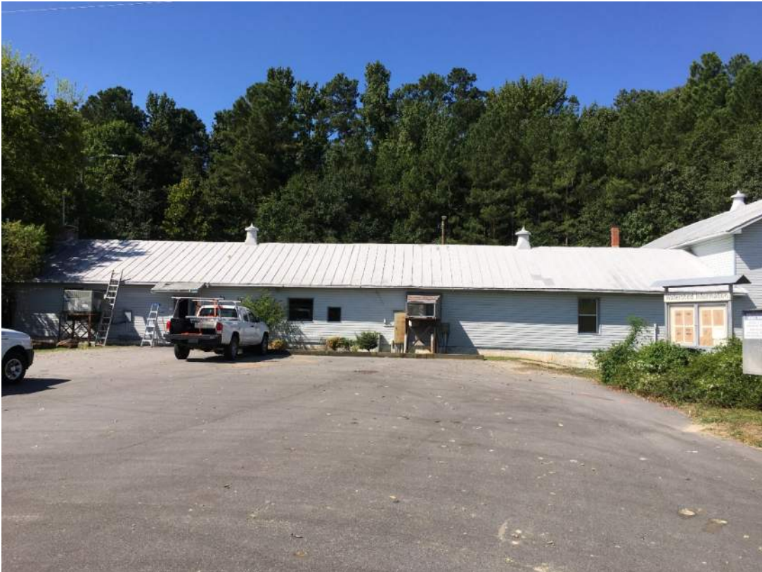
Photo 2: Former WTP Building Southeastern Exterior, Viewed from East
