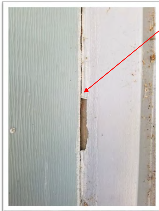
Photograph #0002 Close view of typical Exterior Window Caulking
