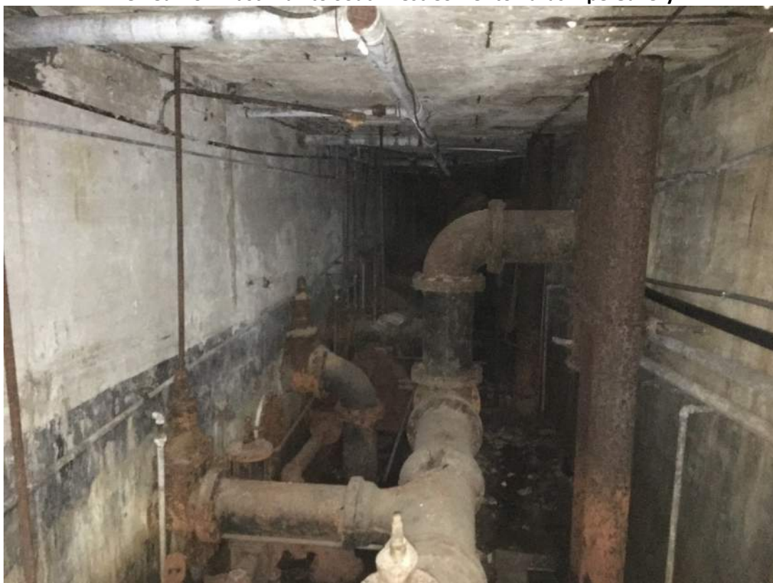
Photo 38: Pipe Gallery Viewed from Opening Beneath Mezzanine to South
