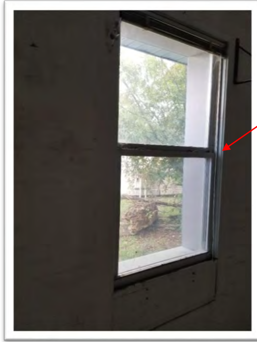
Photograph #0003 White Lead-Based Paint associated with wood window casing in South Room
