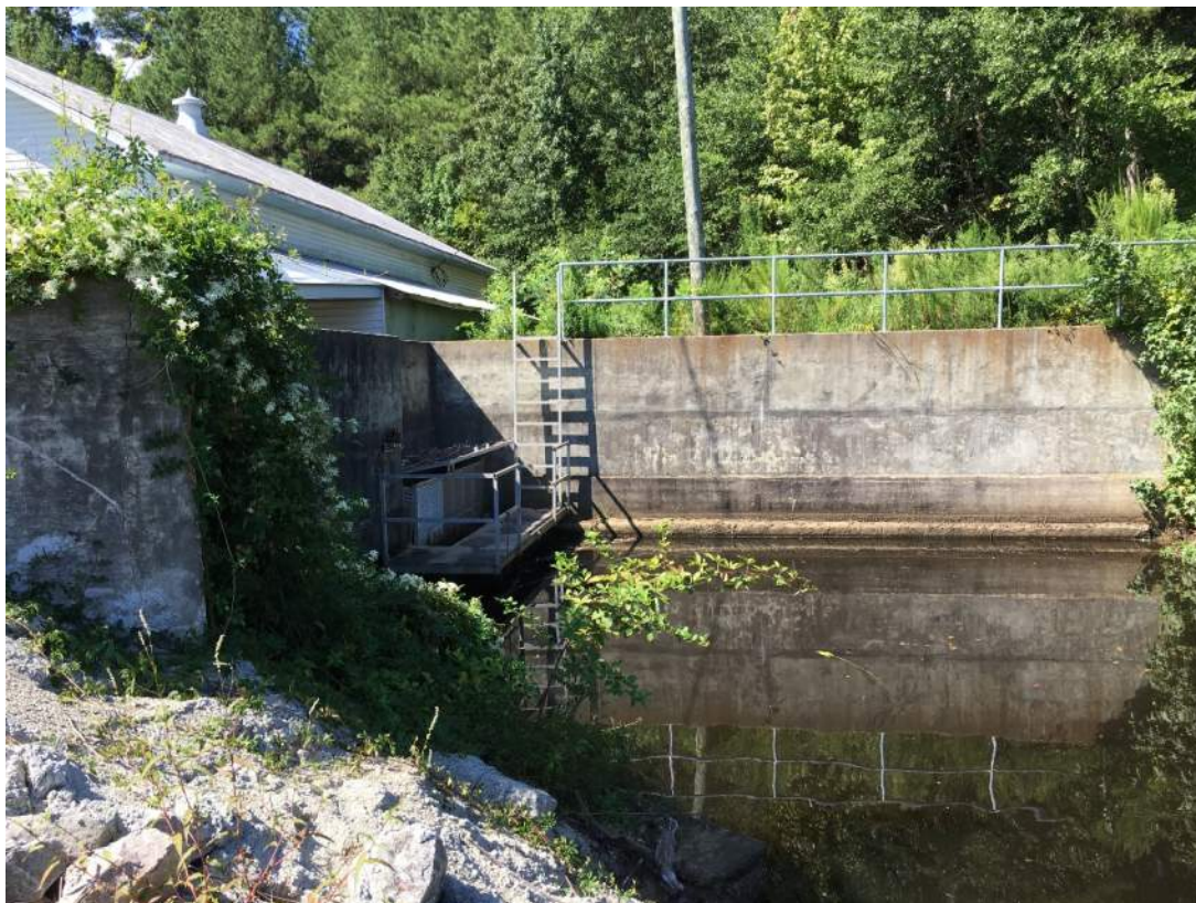
Photo 13: Intake Area and Retaining Wall, Viewed from Dam Upstream Slope
