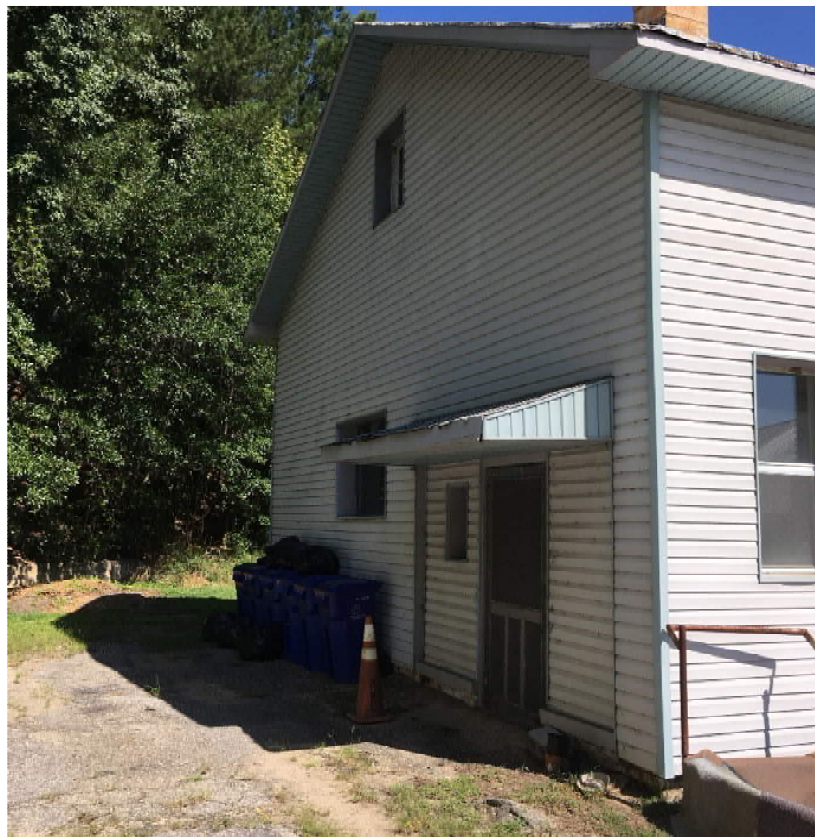
Photo 6: Former WTP Building Northwestern Exterior, Viewed from Northwest
