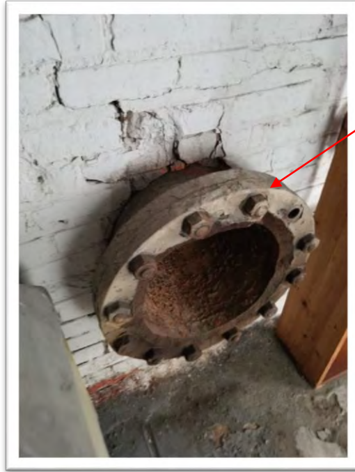
Photograph #0015 Off-White Lead-Based Paint associated with metal pipe in Storage #2
