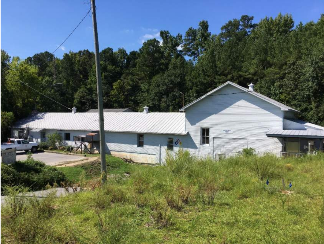
Photo 1: Former WTP Building Eastern Exterior, Viewed from Northeast
