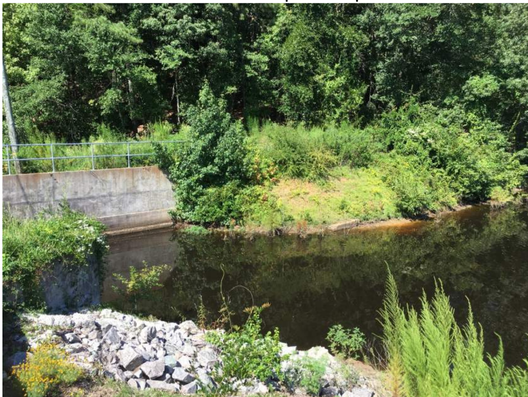
Photo 14: Intake Area, Viewed from Dam Upstream Slope
