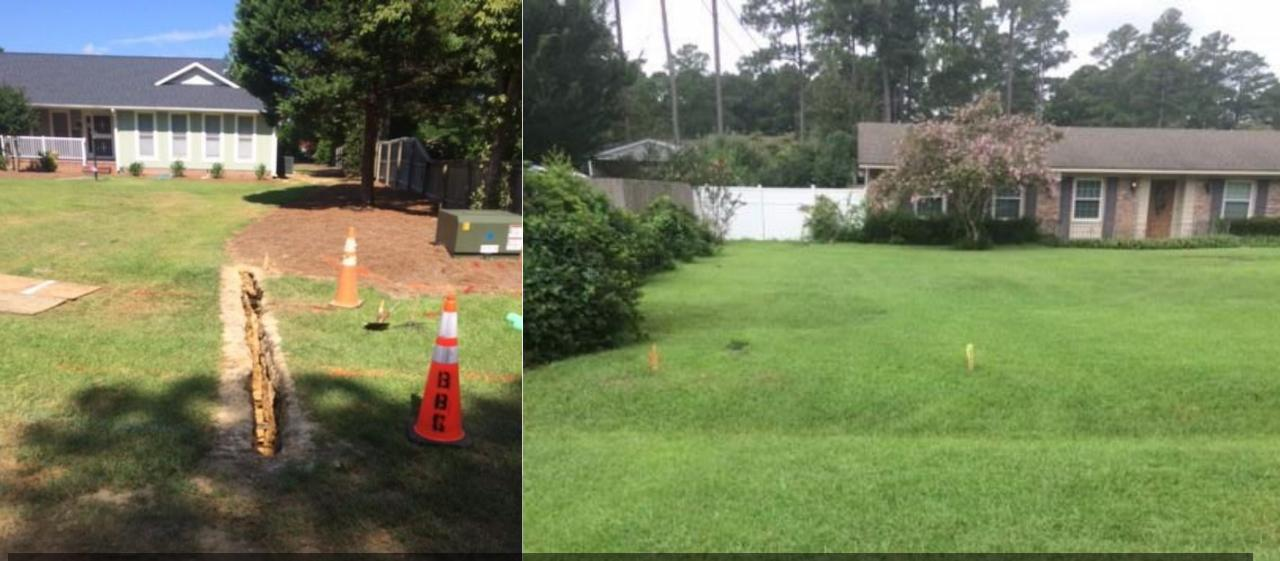
Work will include installation of sewer laterals at each property. Lateral will be installed in the right-of-way/up to your property line. Location of Lateral will be shown on the street/curb.
