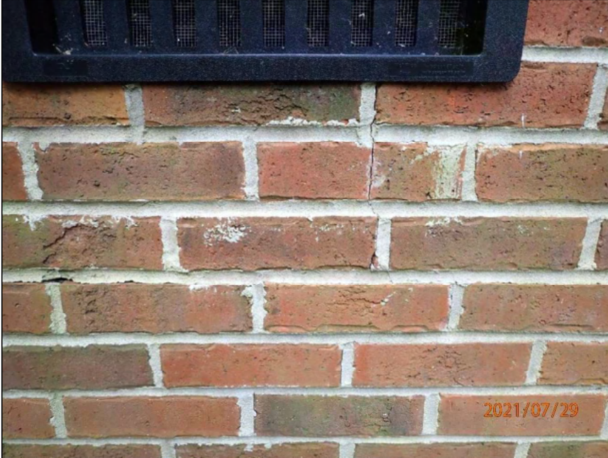
Photo 11 Vertical crack
