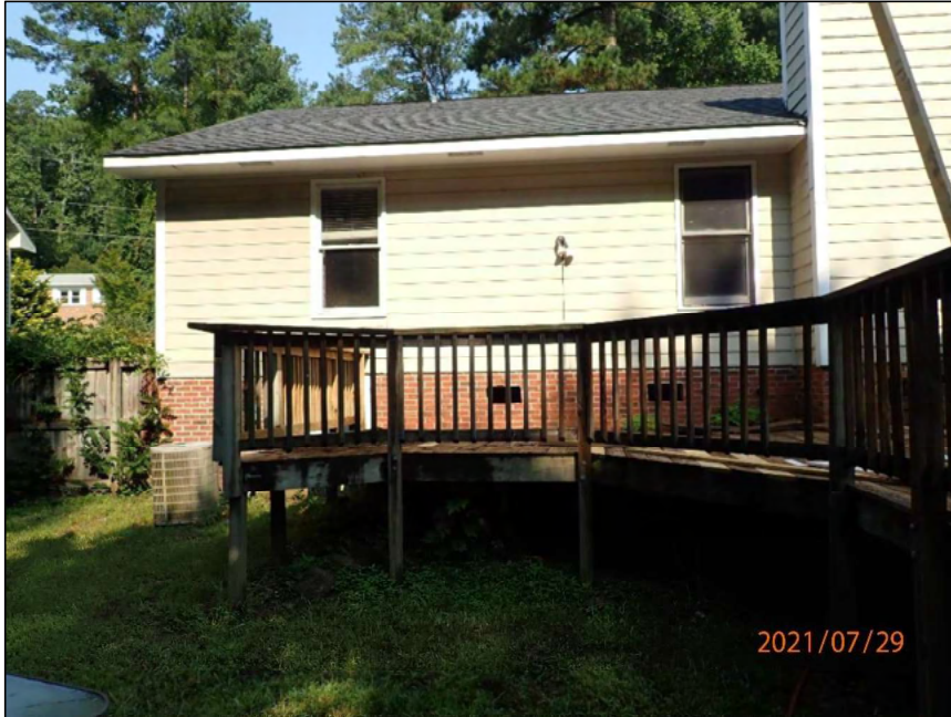
Photo 3 Area of residence observed – rear elevation
