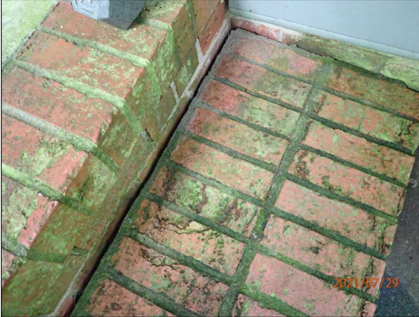
Photo 9 Separation cracks
