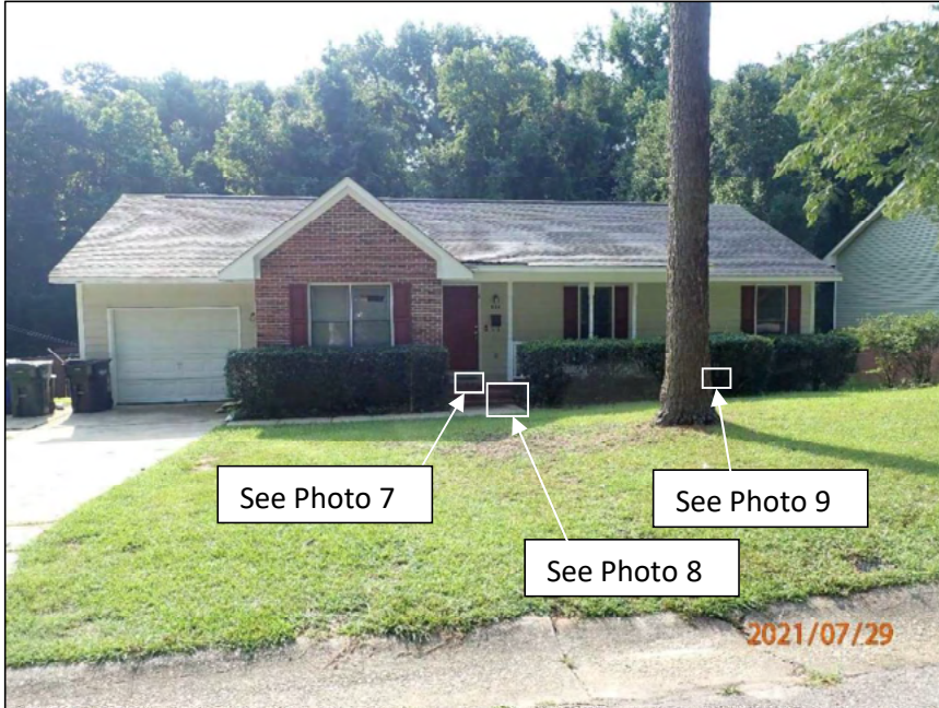
Photo 1 Area of residence observed – front elevation
