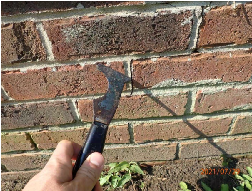
Photo 10 Step crack
