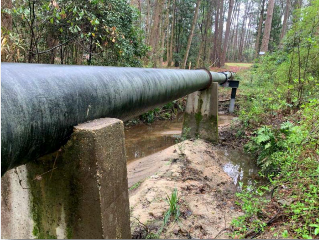
3. View of existing aerial sewer pipe crossing S1 to be replaced.
