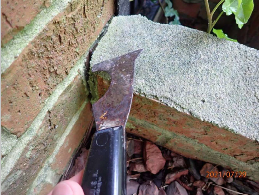
Photo 7 Separation crack
