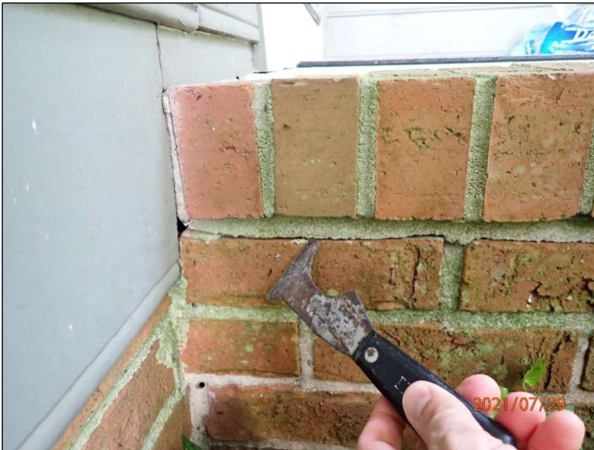
Photo 8 Horizontal crack
