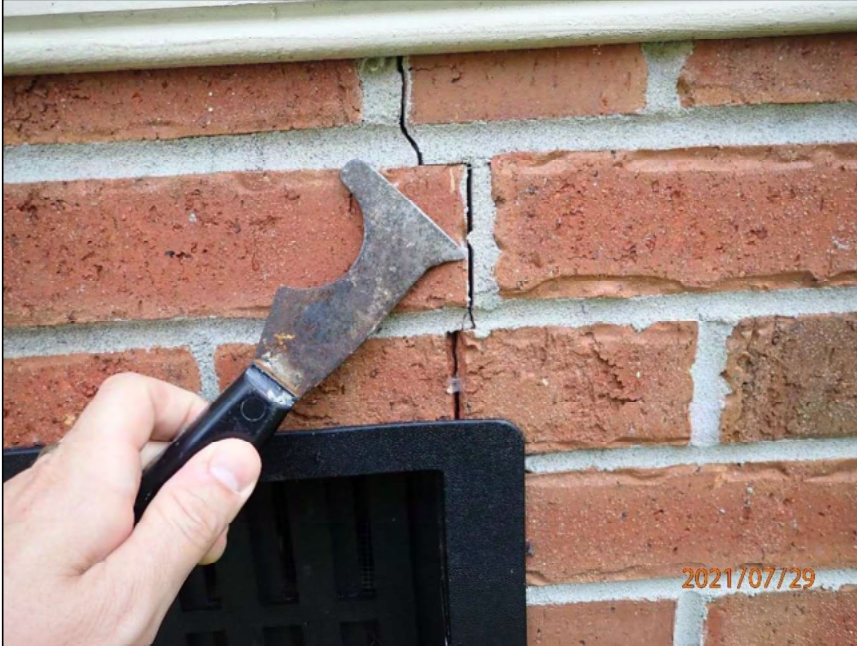
Photo 11 Vertical crack
