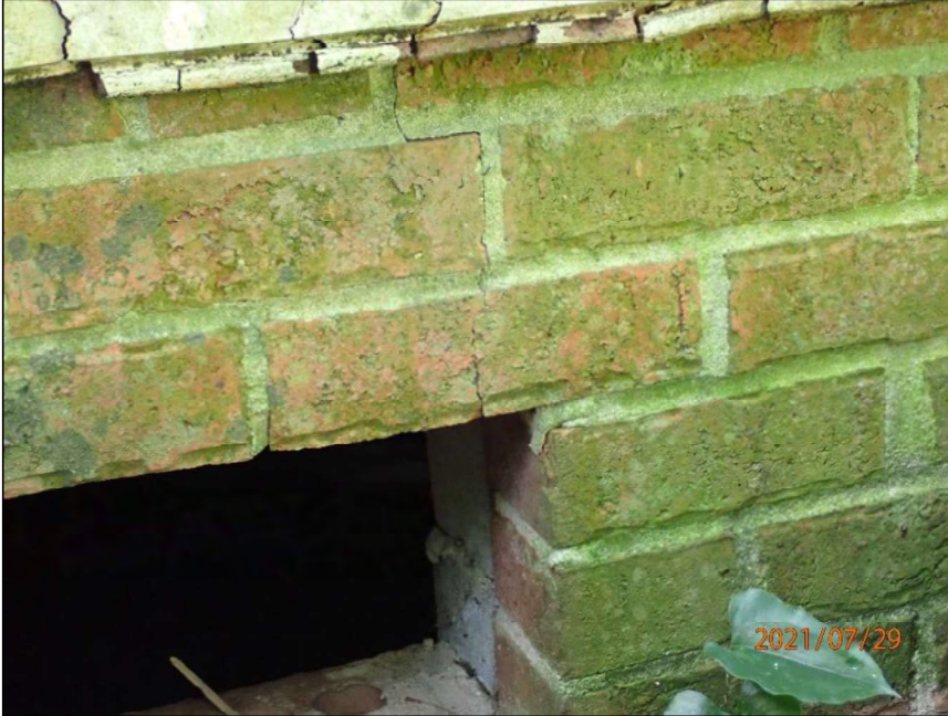
Photo 9 Vertical crack
