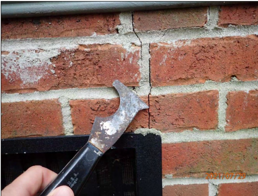
Photo 10 Vertical crack
