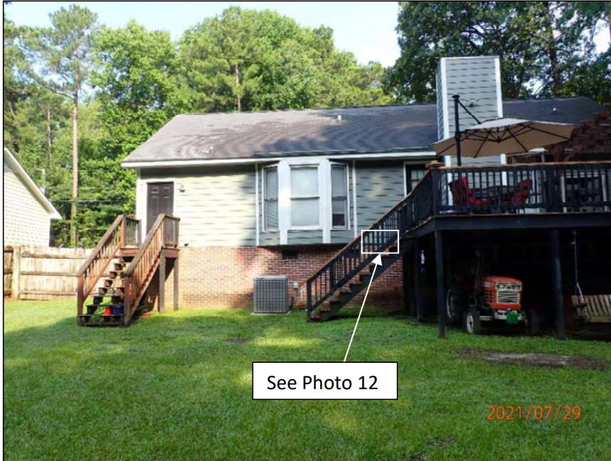
Photo 3 Area of residence observed – rear elevation
