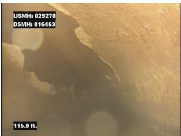
Photo: 029378_D_016463_SAV_115.jpg, VCR No.: 1 115FT, Surface Aggregate Visible, from 08 to 04 o'clock, within 8 inches of joint: NO, Start
