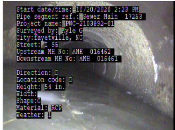
Photo: PWC-2103892-01-AMH '016462'-AMH '016461'-MWL at 0.0 ft.JPG OFT, Water Level, 35% of cross sectional area
