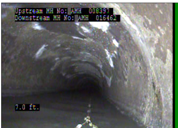
Photo: 008397_D_016462_SAV_7_23_A.jpg, 00:00:33 7FT, Surface Aggregate Visible, from 08 to 04 o'clock, within 8 inches: NO
