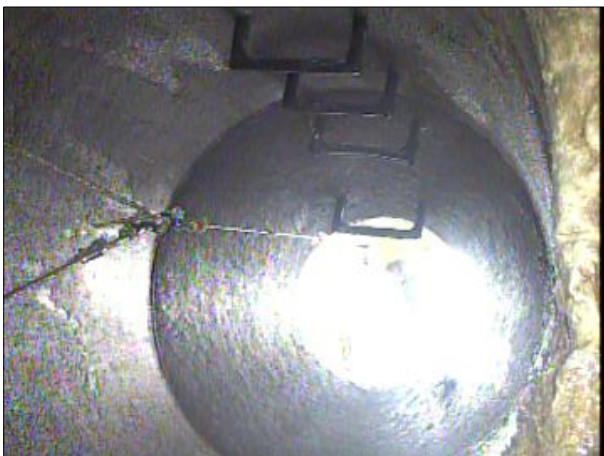
Photo: PWC-2103892-01-AMH '008397'-AMH '016462'-AMH at 374.3 ft.JPG, 00:23:35 374.3FT, Manhole
