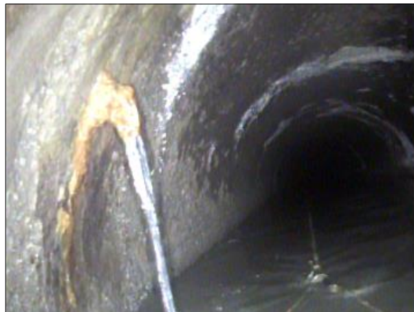
Photo: PWC-2103892-01-AMH '016462'-AMH '016461'-IR at 259.1 ft.JPG, 00:11:50 259.1FT, Infiltration Runner, at 09 o'clock, within 8 inches: NO
