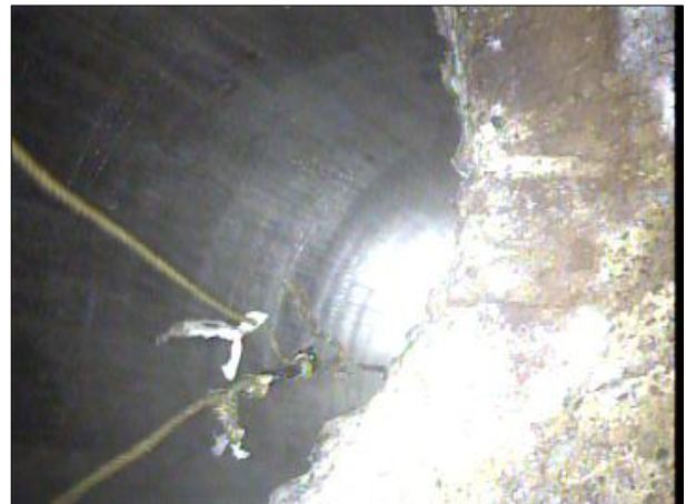
Photo: PWC-2103892-01-AMH '016462'-AMH '016461'-AMH at 792.2 ft.JPG, 00:46:53 792.2FT, Manhole
