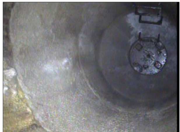
Photo: PWC-2103892-01-AMH '016463'-AMH '008396'-AMH at 848.9 ft.JPG, 03:08:54 848.9FT, Manhole
