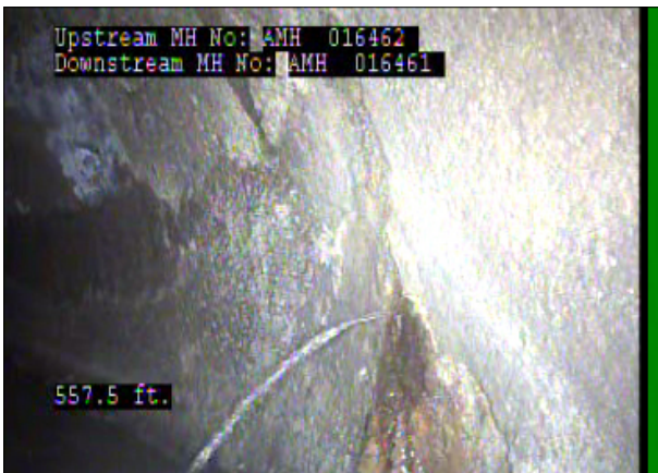
Photo: 016462_D_016461_IR_557.5_43_A.jpg, 00:31:52 557.5FT, Infiltration Runner, at 03 o'clock, within 8 inches: NO
