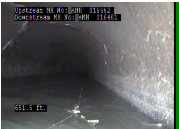
Photo: 016462_D_016461_SRI_651.5_45_A.jpg, 00:37:19 651.5FT, Surface Roughness Increased, from 08 to 04 o'clock, within 8 inches: NO
