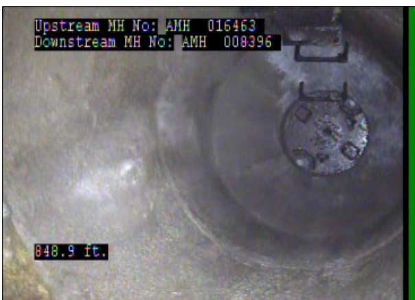
Photo: 016463_D_008396_AMH_848.9_5_A.jpg, 03:08:54 848.9FT, Manhole
