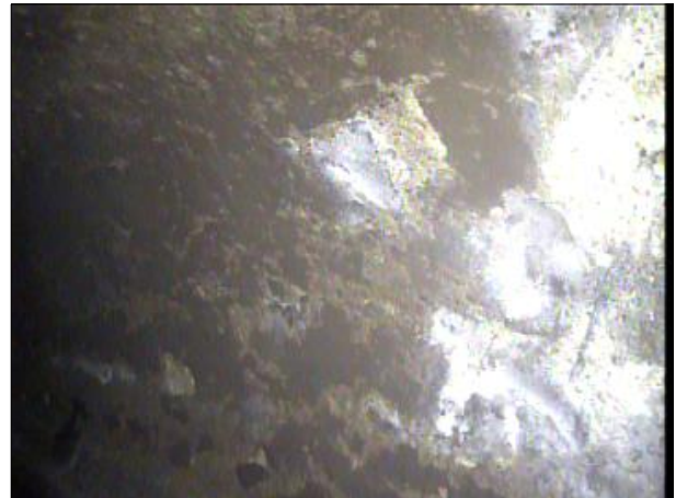
Photo: PWC-2103892-01-AMH '016462'-AMH '016461'-MGP at 58.4 ft.JPG, 00:02:39 58.4FT, General Photograph
