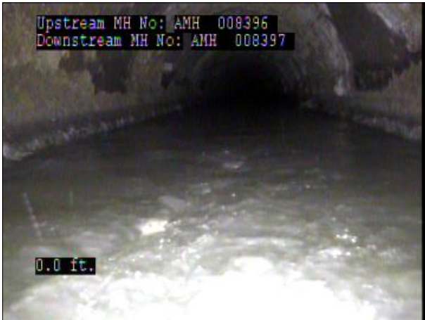
Photo: PWC-2103892-01-AMH '008396'-AMH '008397'-AMH at 0.0 ft.JPG 0FT, Manhole
