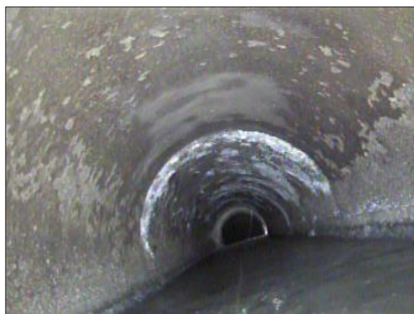
Photo: PWC-2103892-01-AMH '008396'-AMH '008397'-SAV at 587.5 ft.JPG, 00:32:23 587.5FT, Surface Aggregate Visible, from 09 to 03 o'clock, within 8 inches: NO
