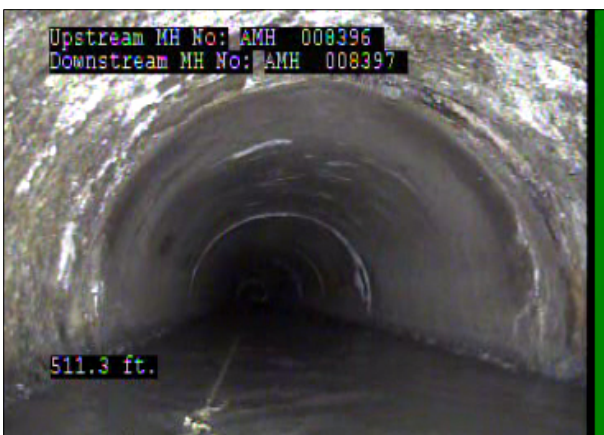
Photo: 008396_D_008397_SAP_511.4_16_A.jpg, 00:27:08 511.4FT, Surface Aggregate Projecting, from 09 to 03 o'clock, within 8 inches of joint: NO, Finish
