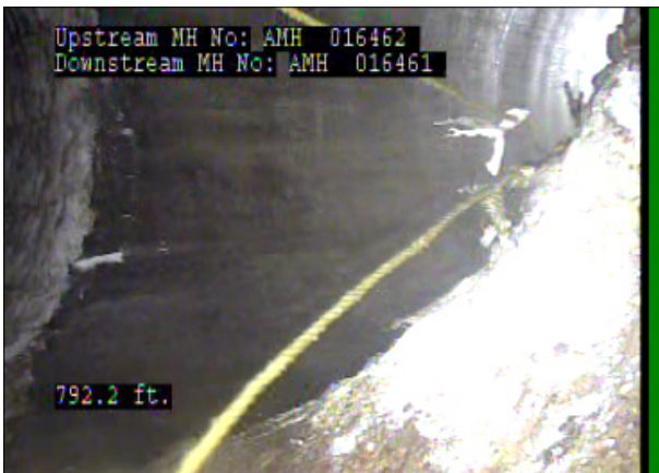
Photo: 016462_D_016461_AMH_792.2_49_A.jpg, 00:46:53 792.2FT, Manhole
