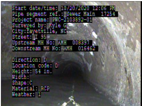
Photo: PWC-2103892-01-AMH '008397'-AMH '016462'-AMH at 0.0 ft.JPG OFT, Manhole
