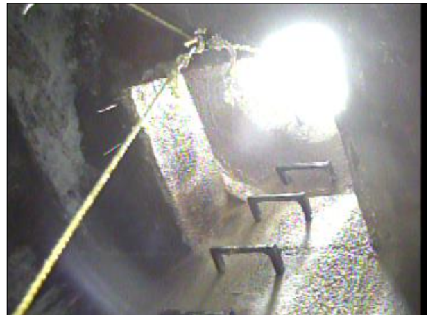
Photo: PWC-2103892-01-AMH '008396'-AMH '008397'-AMH at 636.7 ft.JPG, 00:35:50 636.7FT, Manhole
