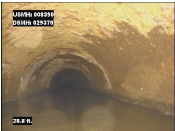
Photo: 008390_D_029378_SAV_28.8.jpg, VCR No.: 1 28.8FT, Surface Aggregate Visible, from 08 to 04 o'clock, within 8 inches of joint: NO, Start
