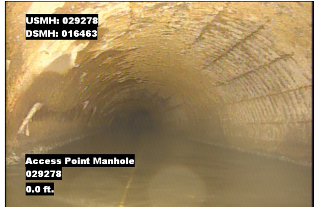
Photo: 029378_D_016463_AMH_0.jpg, VCR No.: 1 0FT, Manhole
