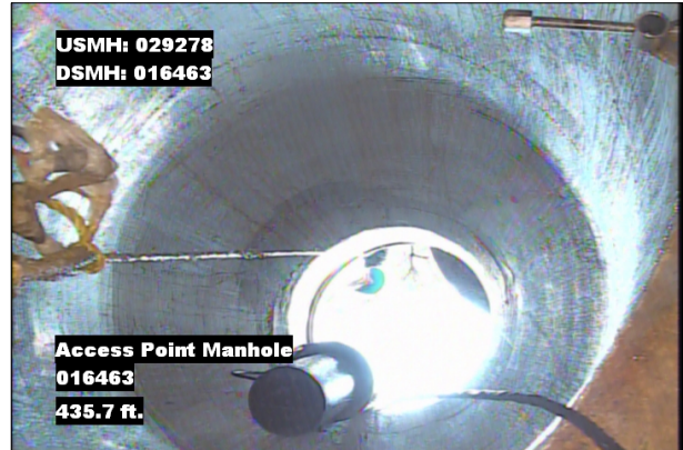
Photo: 029378_D_016463_AMH_435.7.jpg, VCR No.: 1 435.7FT, Manhole
