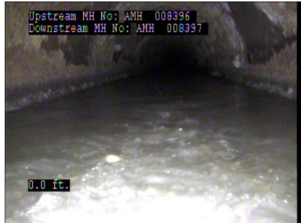
Photo: PWC-2103892-01-AMH '008396'-AMH '008397'-MWL at 0.0 ft.JPG 0FT, Water Level, 30 %of cross sectional area
