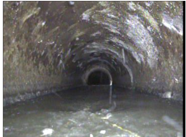
Photo: PWC-2103892-01-AMH '008396'-AMH '008397'-SRI at 599.3 ft.JPG, 00:33:38 599.3FT, Surface Roughness Increased, from 09 to 03 o'clock, within 8 inches: NO
