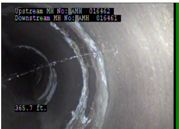
Photo: 016462_D_016461_IR_365.7_37_A.jpg, 00:18:26 365.7FT, Infiltration Runner, at 12 o'clock, within 8 inches: NO
