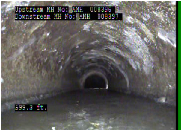
Photo: 008396_D_008397_SRI_599.3_19_A.jpg, 00:33:38 599.3FT, Surface Roughness Increased, from 09 to 03 o'clock, within 8 inches: NO
