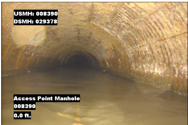
Photo: 008390_D_029378_AMH_0.jpg, VCR No.: 1 0FT, Manhole
