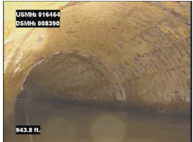
Photo: 016464_D_008390_LL_943.jpg, VCR No.: 1 943FT, Alignment Left, 20 %
