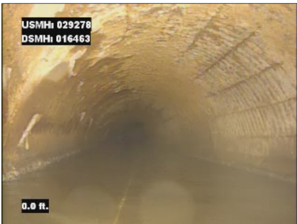
Photo: 029378_D_016463_SRV_1.jpg, VCR No.: 1 1FT, Surface Reinforcement Visible, from 08 to 04 o'clock, within 8 inches of joint: NO, Start
