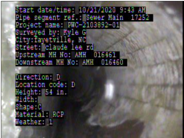
Photo: PWC-2103892-01-AMH '016461'-AMH '016460'-AMH at 0.0 ft.JPG OFT, Manhole
