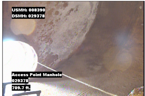
Photo: 008390_D_029378_AMH_709.7.jpg, VCR No.: 1 709.7FT, Manhole
