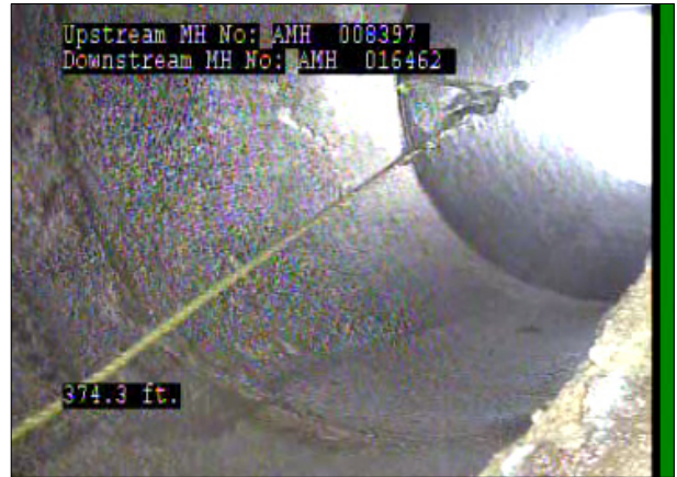
Photo: 008397_D_016462_AMH_374.3_30_A.jpg, 00:23:35 374.3FT, Manhole
