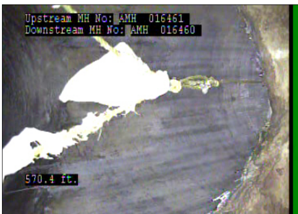
Photo: 016461_D_016460_AMH_570.4_57_A.jpg, 00:30:09 570.4FT, Manhole
