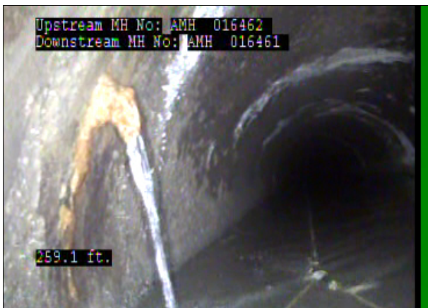
Photo: 016462_D_016461_IR_259.1_36_A.jpg, 00:11:50 259.1FT, Infiltration Runner, at 09 o'clock, within 8 inches: NO
