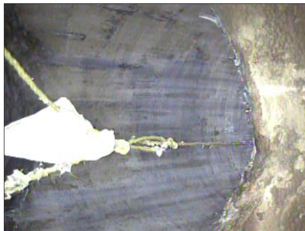
Photo: PWC-2103892-01-AMH '016461'-AMH '016460'-AMH at 570.4 ft.JPG, 00:30:09 570.4FT, Manhole
