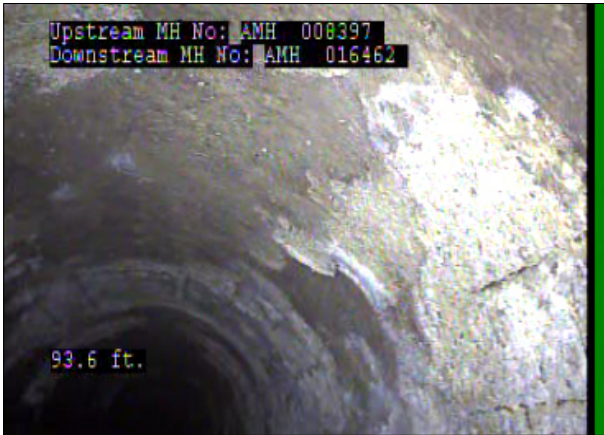
Photo: 008397_D_016462_SAV_93.4_24_A.jpg, 00:04:11 93.4FT, Surface Aggregate Visible, from 08 to 04 o'clock, within 8 inches: NO
