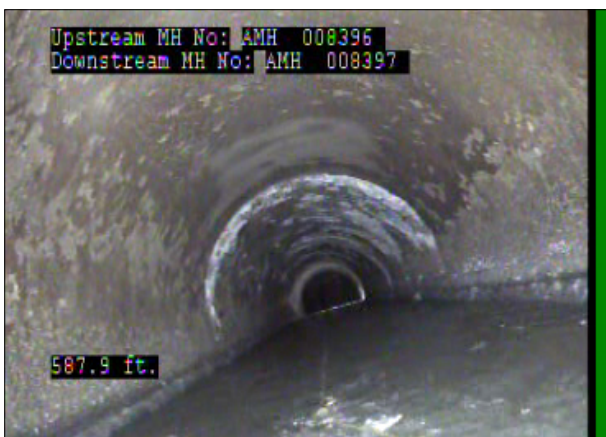
Photo: 008396_D_008397_SAV_587.5_18_A.jpg, 00:32:23 587.5FT, Surface Aggregate Visible, from 09 to 03 o'clock, within 8 inches: NO
