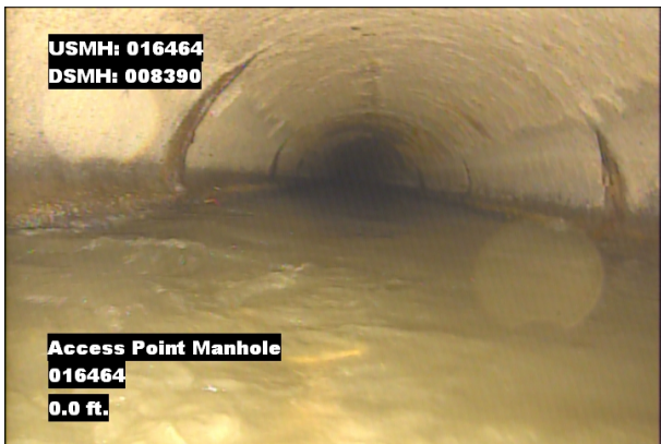
Photo: 016464_D_008390_AMH_0.jpg, VCR No.: 1 0FT, Manhole
