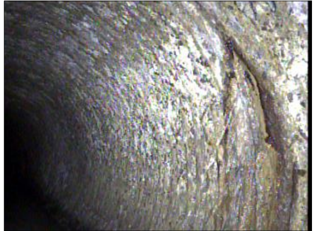
Photo: PWC-2103892-01-AMH '008396'-AMH '008397'-IR at 161.5 ft.JPG, 00:06:41 161.5FT, Infiltration Runner, from 02 to 03 o'clock, within 8 inches: NO
