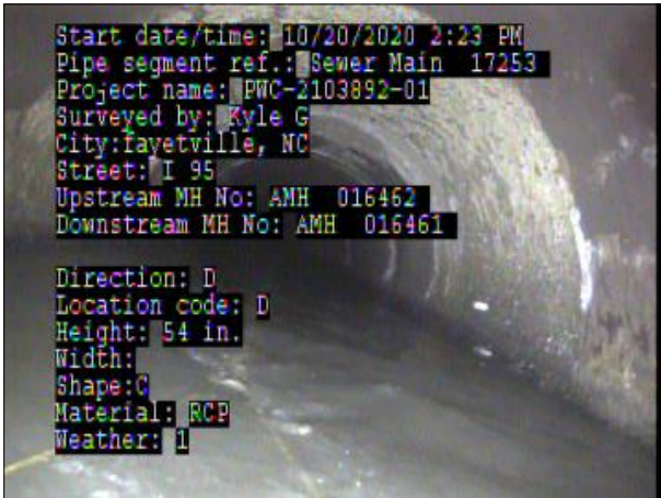
Photo: PWC-2103892-01-AMH '016462'-AMH '016461'-AMH at 0.0 ft.JPG OFT, Manhole
