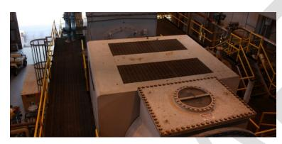
The third component is the Steam Turbines. We conducted a major inspection. The bottom portion is the turbine, where the steam goes in, and the top portion is the generator.
