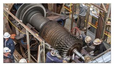
Turbine rotor weighs 23k lbs. A crane has to come to lift the rotor out of the casing. There are about 3 credit cards of clearance.
