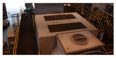
The third component is the Steam Turbines. We conducted a major inspection. The bottom portion is the turbine, where the steam goes in, and the top portion is the generator.
