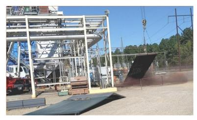
These are the tubes that needed to be replaced. They are about 40 feet and weigh about 40,000 lbs. There were 32 of them in one boiler, for a total of 96.
