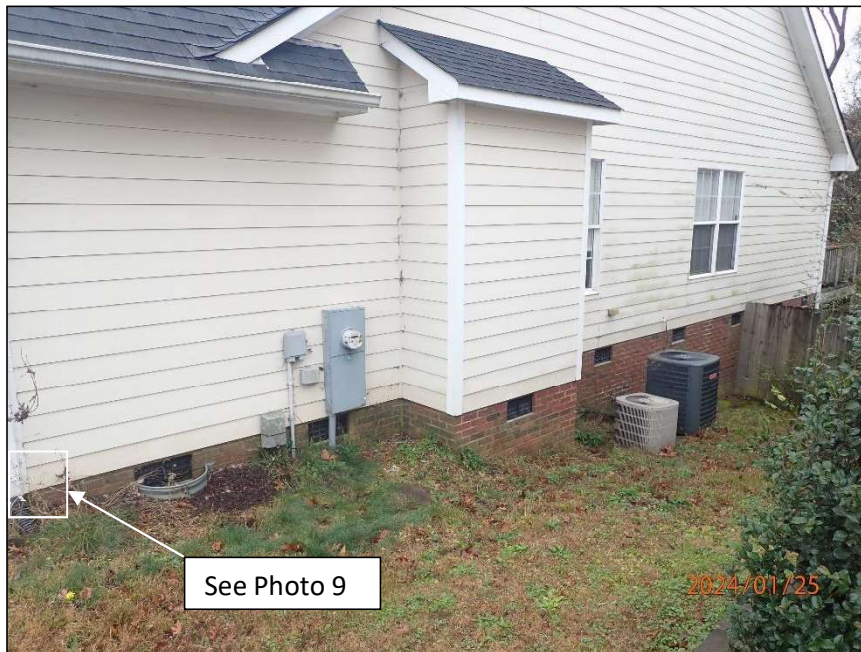
Photo 2 Area of residence observed – side elevation
