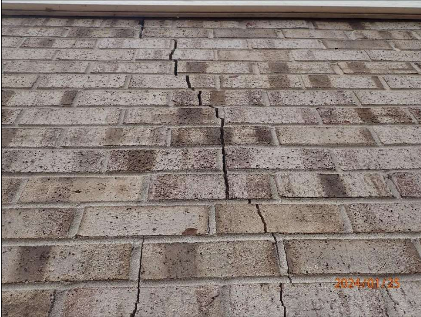
Photo 9 Vertical crack
