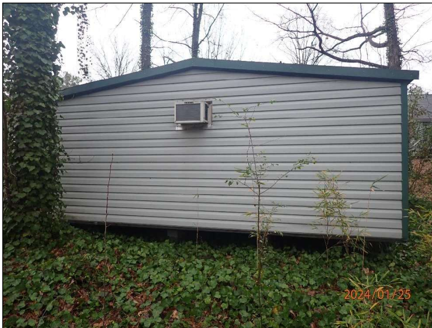
Photo 4 Area of shed observed – back elevation
