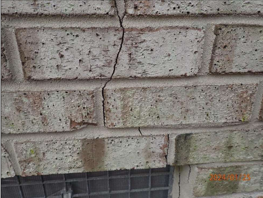
Photo 11 Vertical crack
