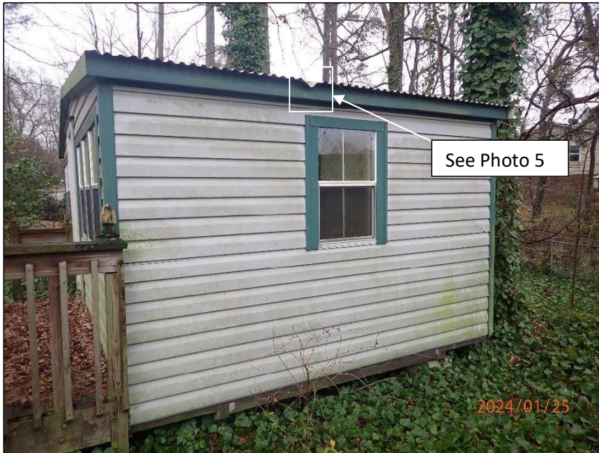
Photo 2 Area of shed observed – side elevation
