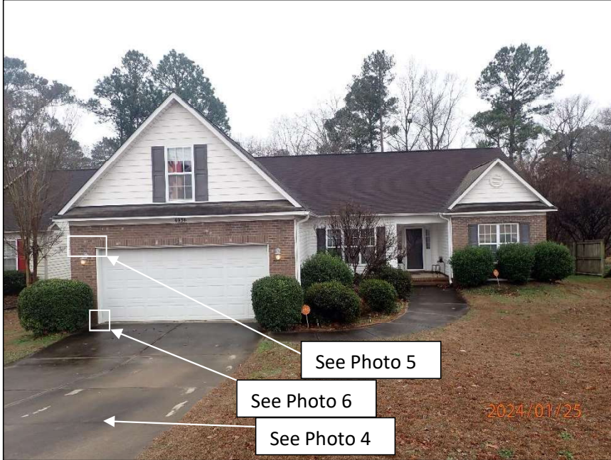
Photo 1 Area of residence observed – front elevation
