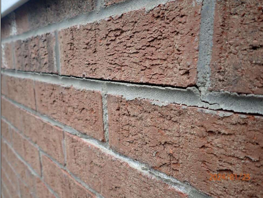
Photo 11 Horizontal crack
