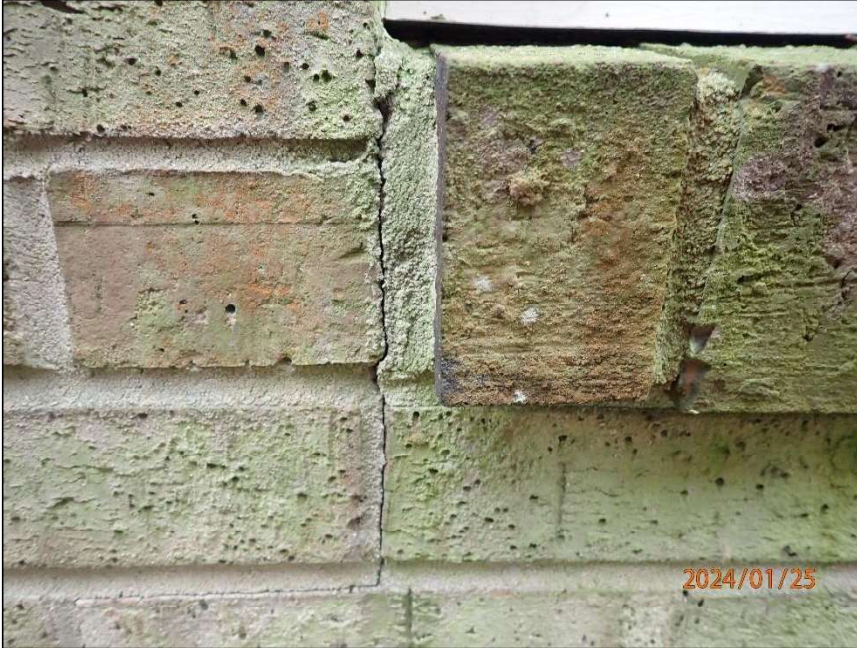
Photo 13 Step crack
