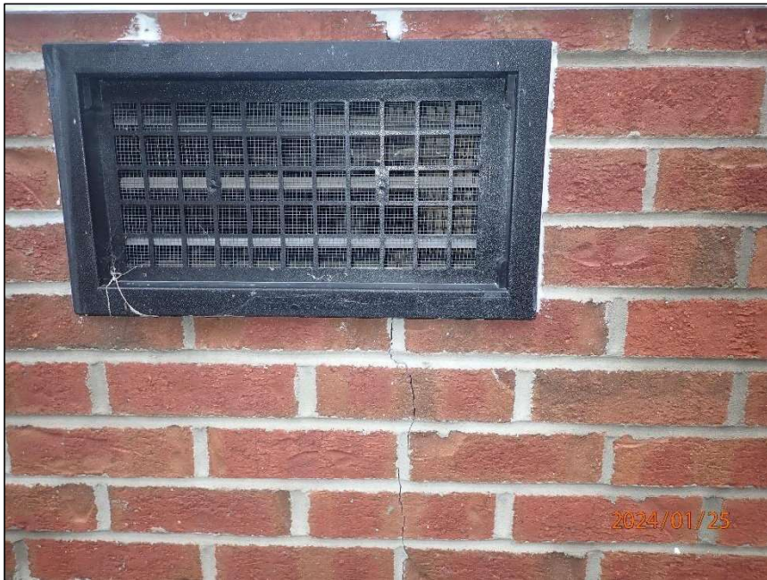
Photo 10 Vertical crack
