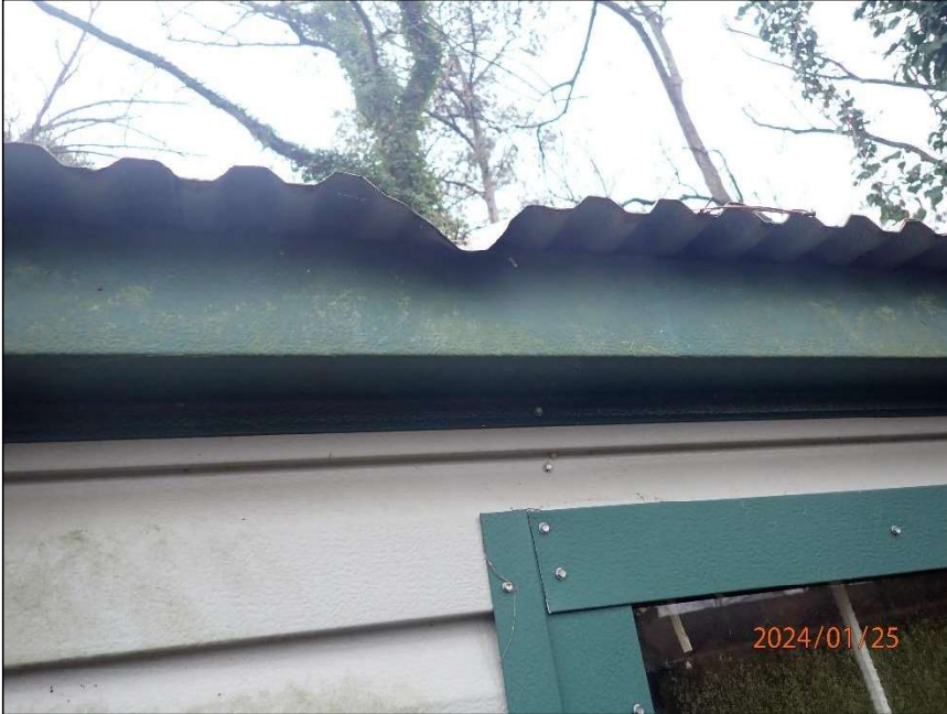
Photo 5 Roof dent
