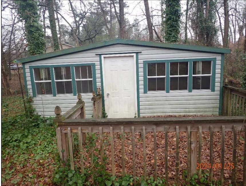
Photo 1 Area of shed observed – front elevation
