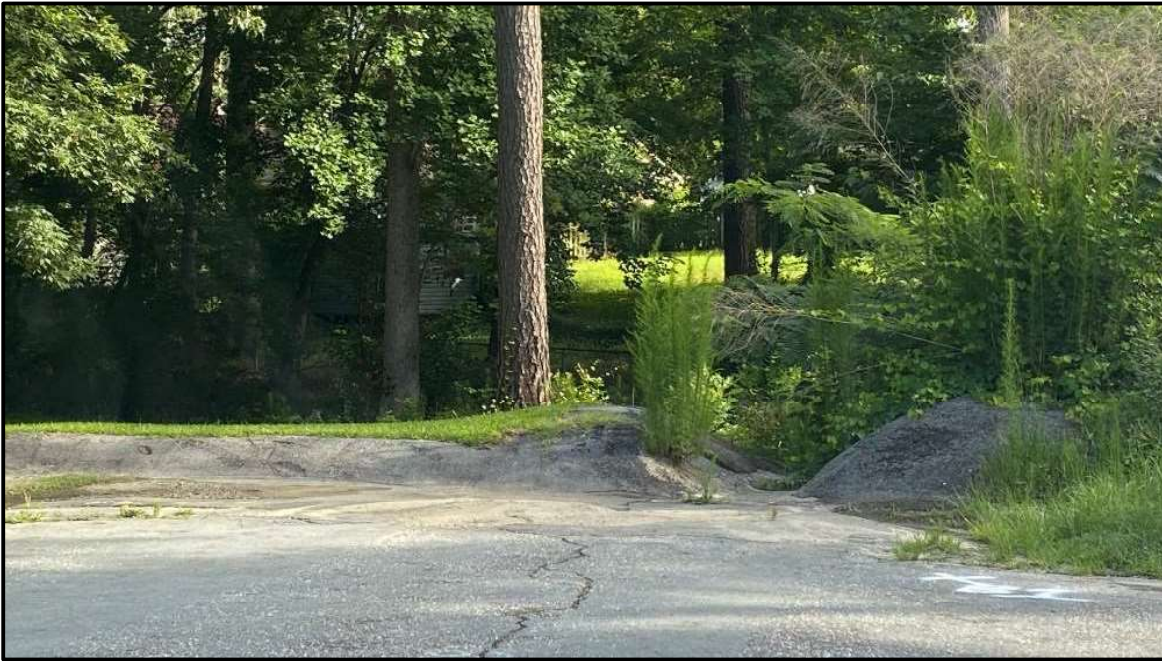
Figure 2: Flume Leading into Creek
