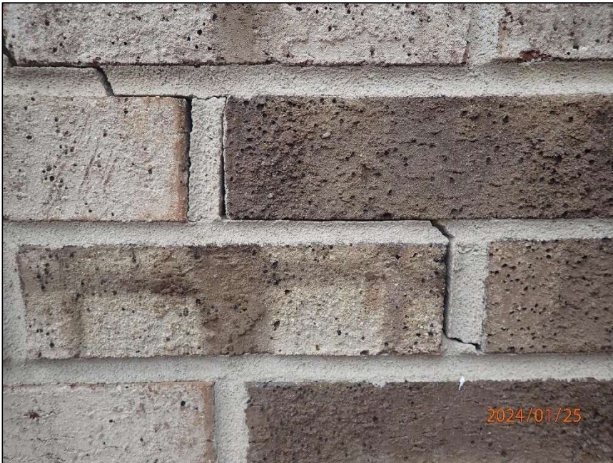
Photo 10 Step crack
