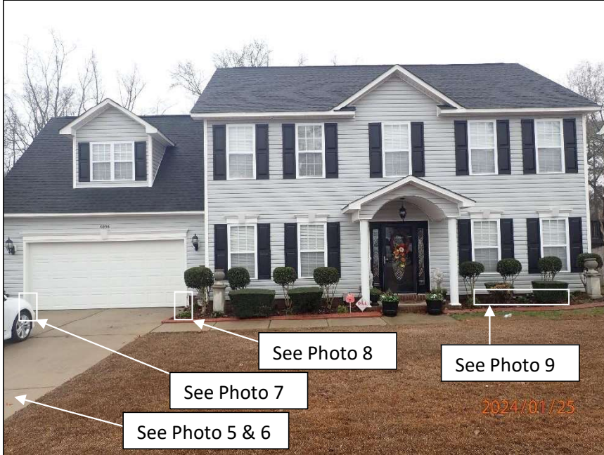
Photo 1 Area of residence observed – front elevation
