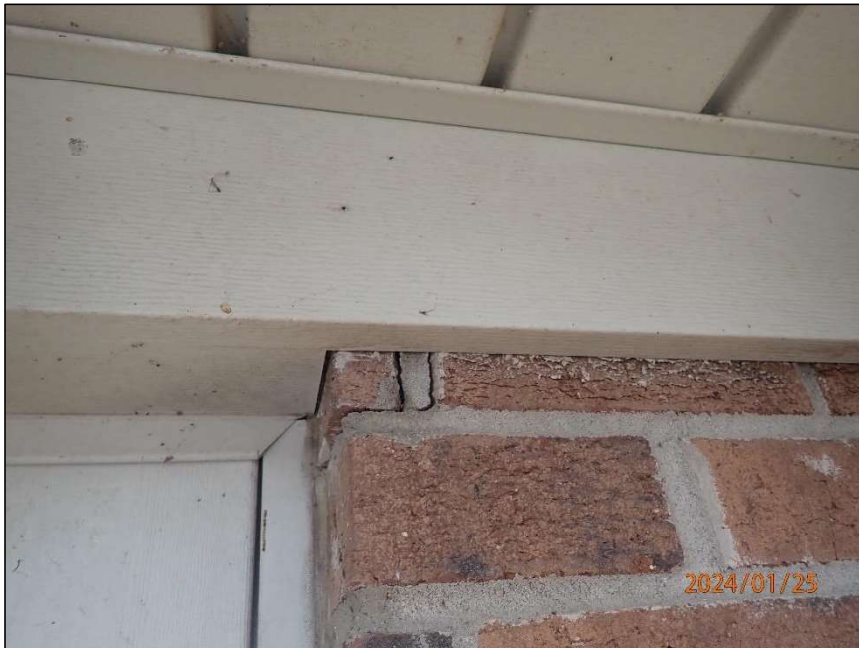
Photo 6 Separation crack
