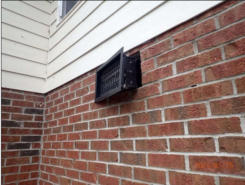
Photo 11 Displaced vent
