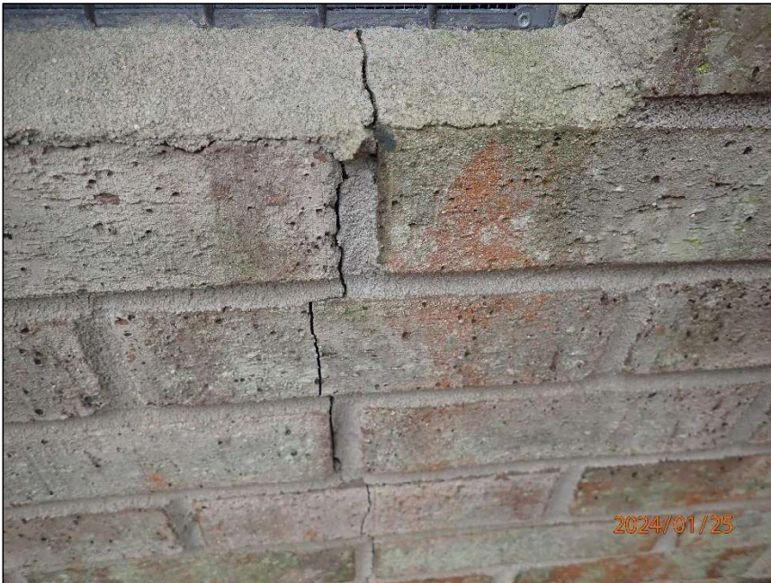
Photo 12 Vertical crack
