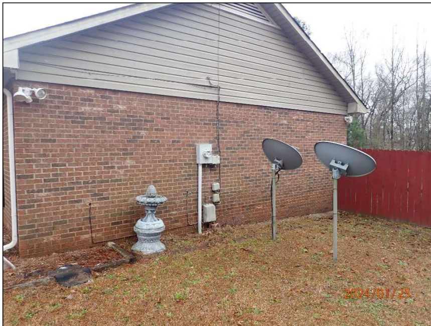
Photo 2 Area of residence observed – side elevation
