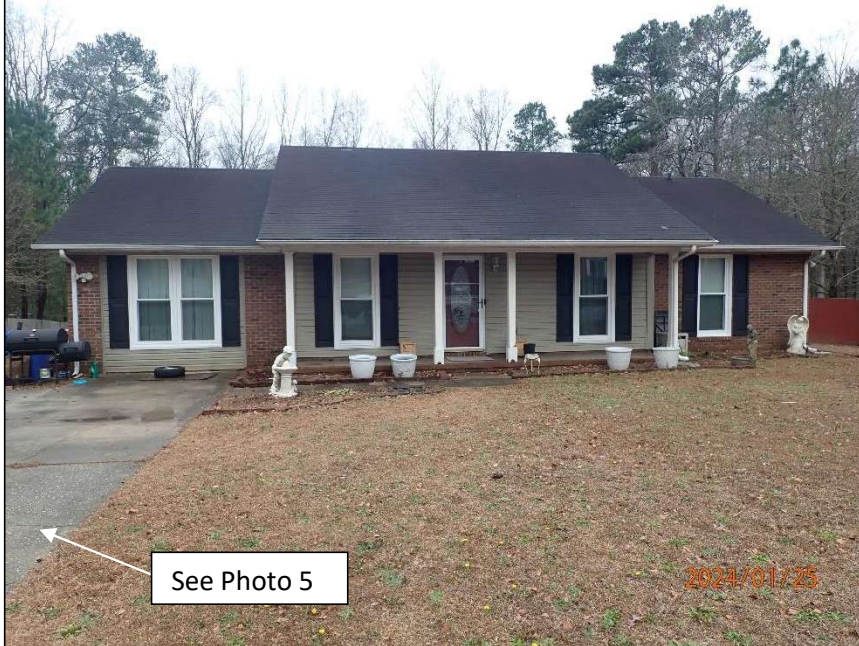
Photo 1 Area of residence observed – front elevation
