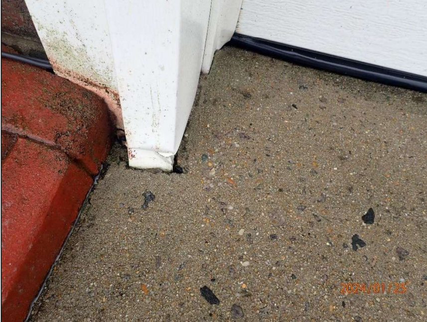
Photo 7 Damaged trim
