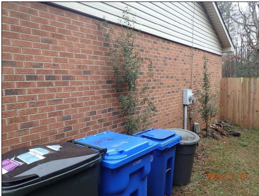
Photo 2 Area of residence observed – side elevation
