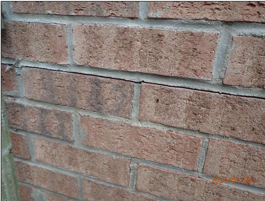
Photo 8 Horizontal crack
