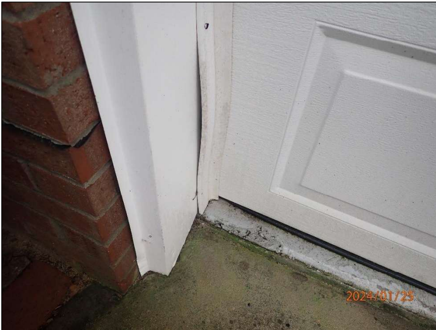
Photo 6 Damaged trim
