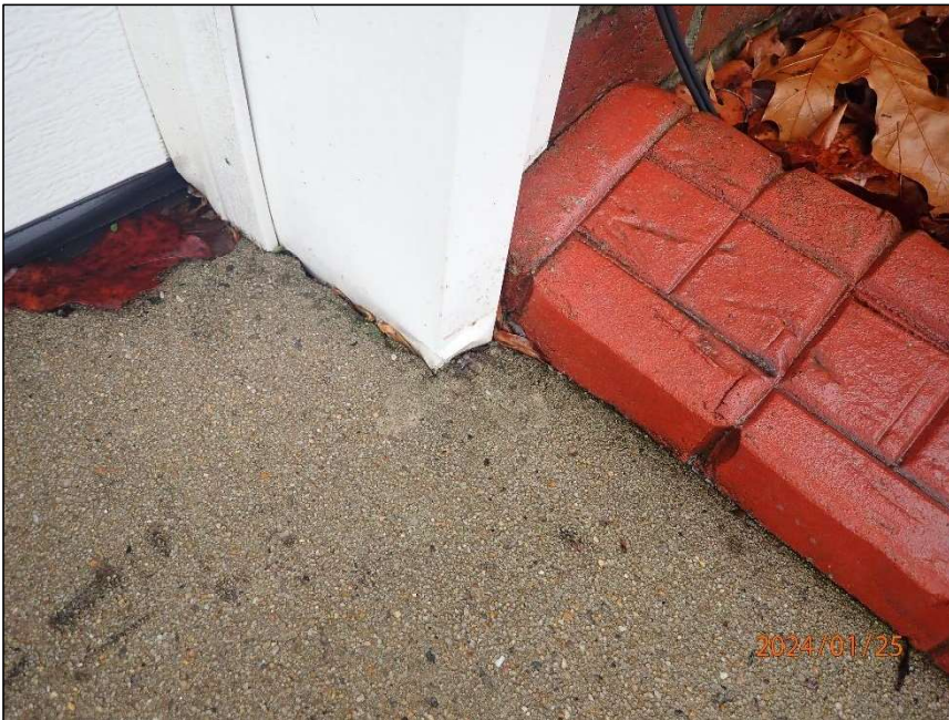
Photo 8 Damaged trim
