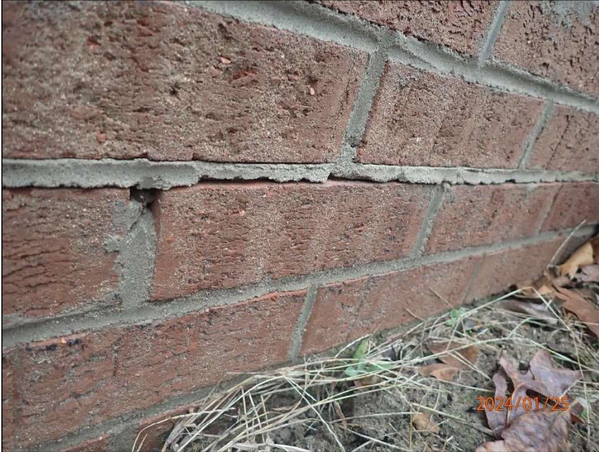
Photo 9 Spalling mortar
