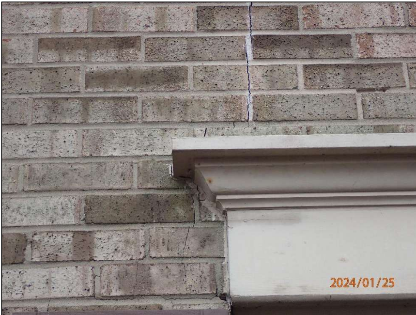
Photo 8 Step crack
