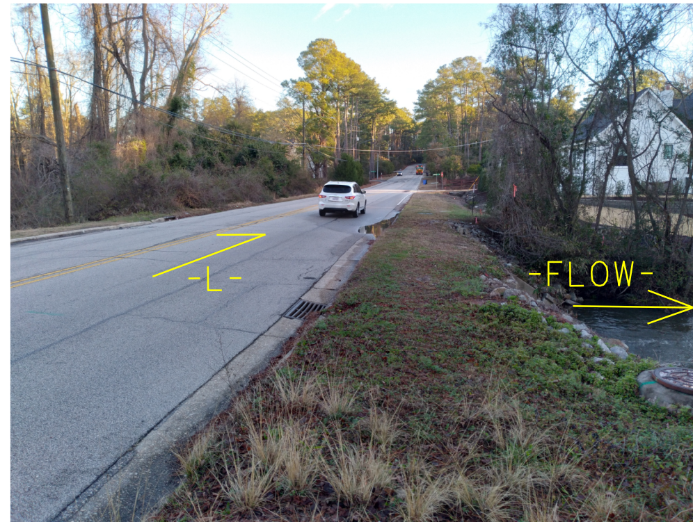
PHOTO #1: END BENT 1 OF EXISTING STRUCTURE NO. 250245 LOOKING NORTHEAST (UPSTATION)
