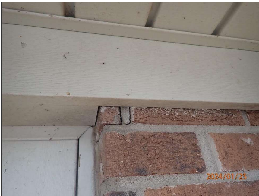
Photo 6 Separation crack
