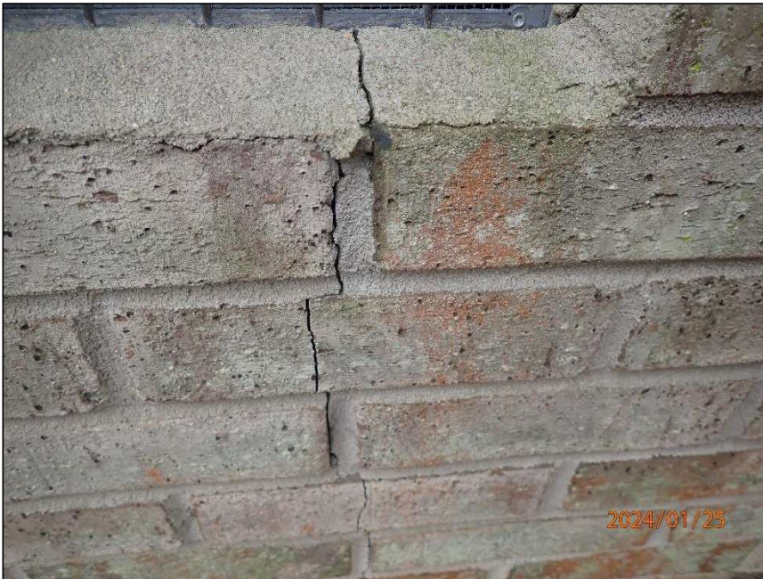
Photo 12 Vertical crack
