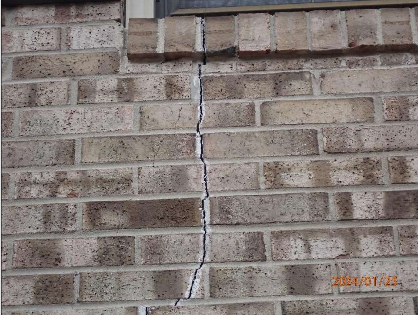
Photo 7 Vertical crack
