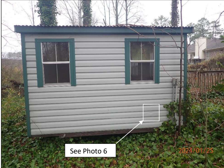
Photo 3 Area of shed observed – side elevation
