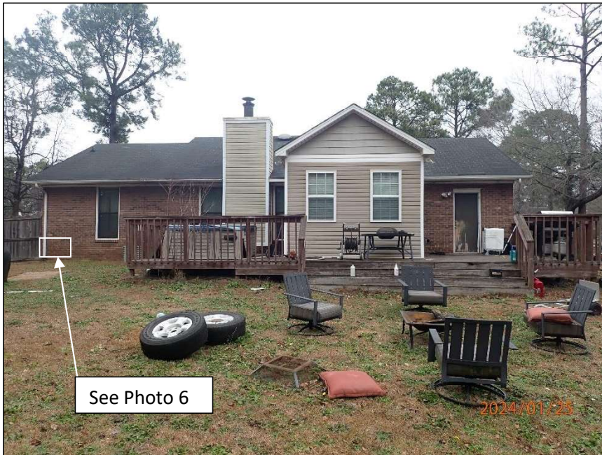
Photo 4 Area of residence observed – back elevation
