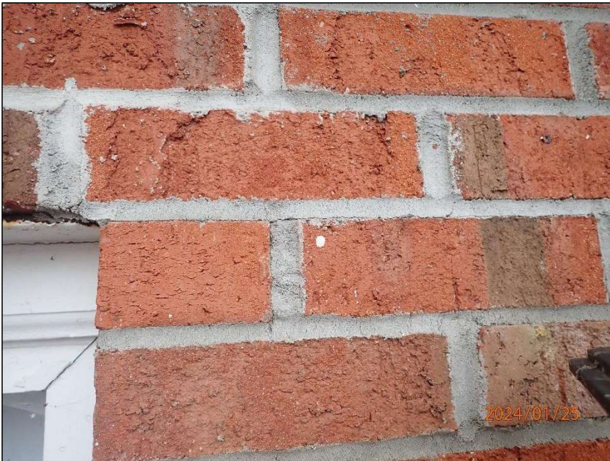
Photo 8 Step crack
