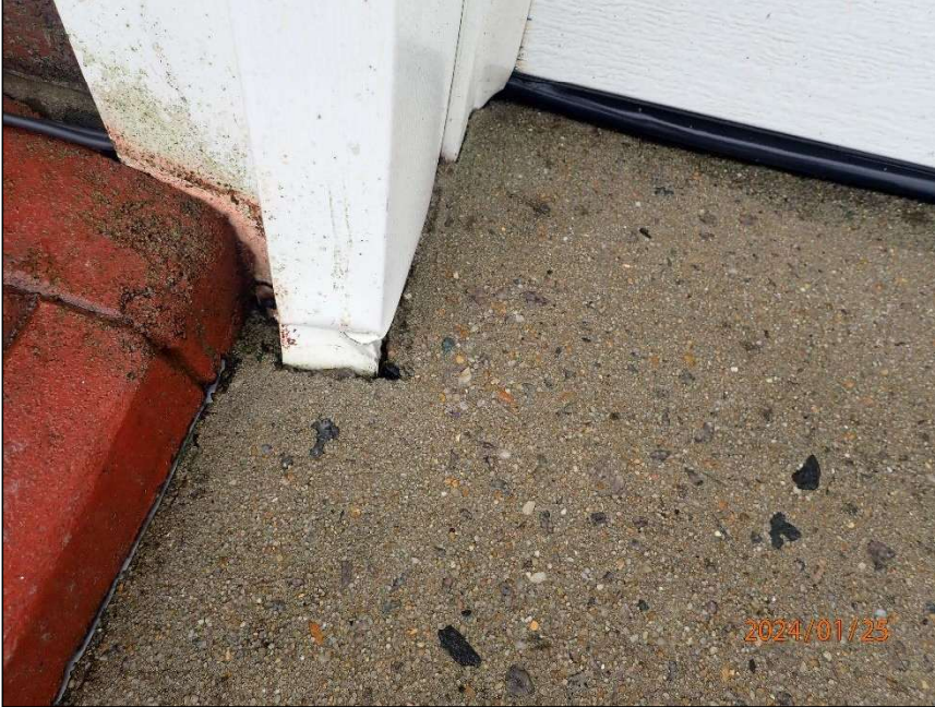
Photo 7 Damaged trim
