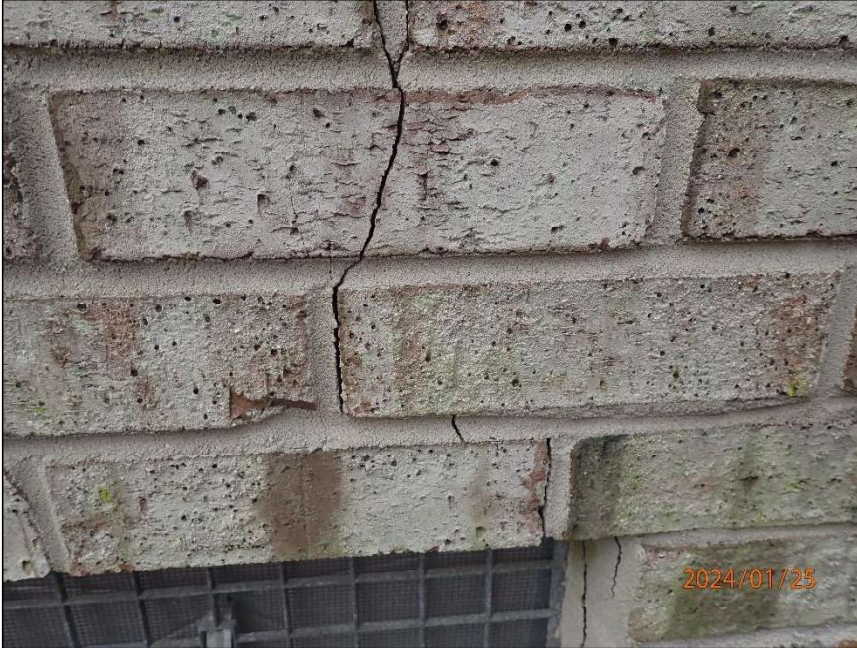
Photo 11 Vertical crack
