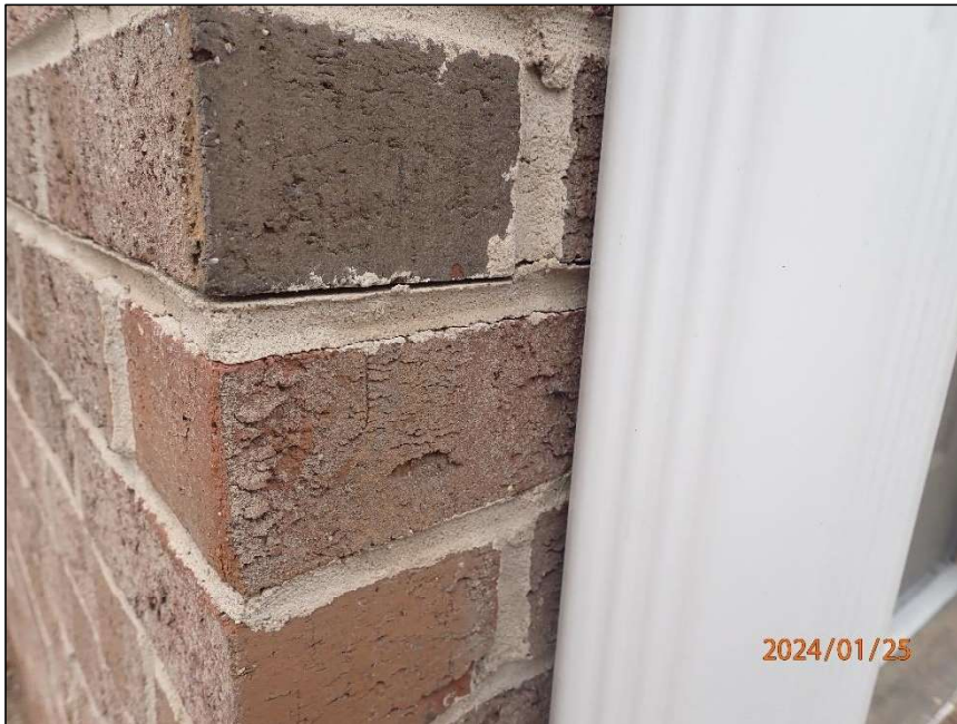
Photo 8 Horizontal crack
