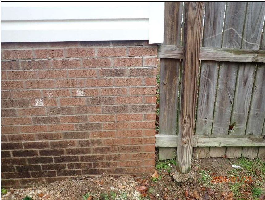
Photo 10 Step crack
