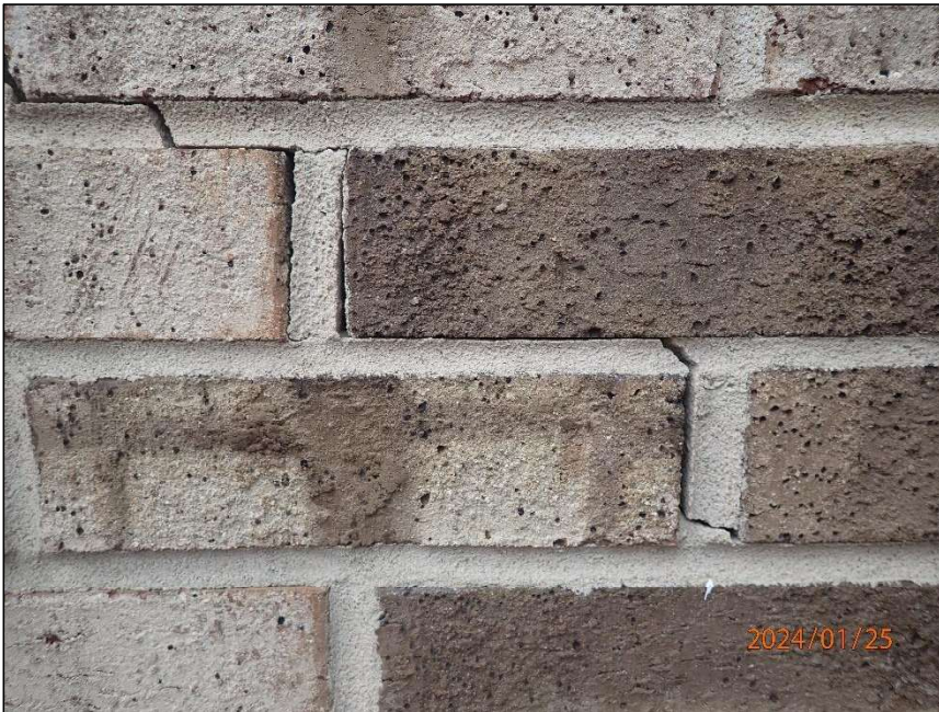
Photo 10 Step crack
