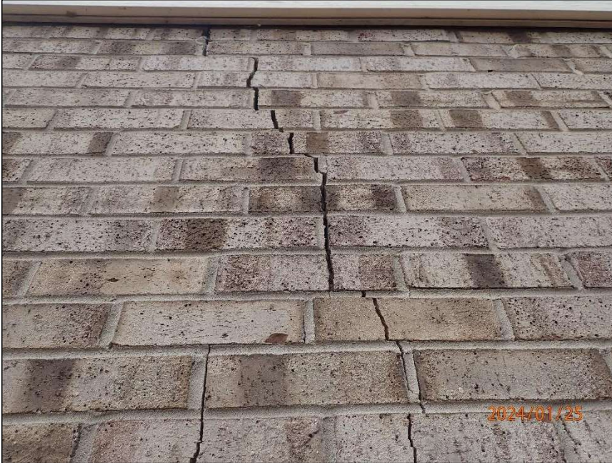
Photo 9 Vertical crack
