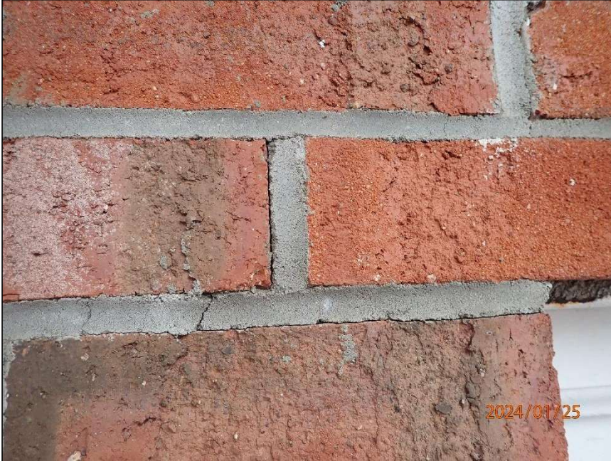
Photo 7 Step crack
