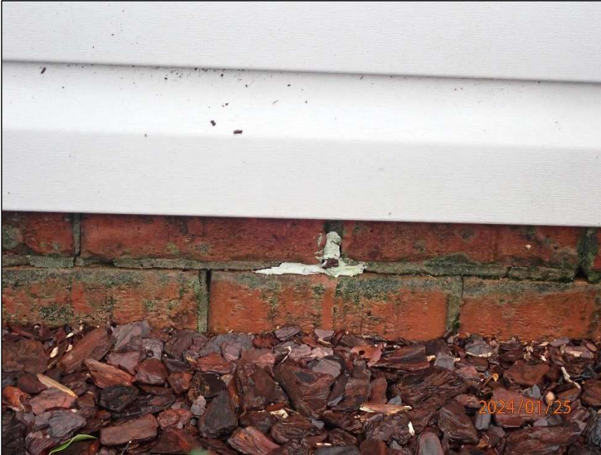
Photo 9 Horizontal crack
