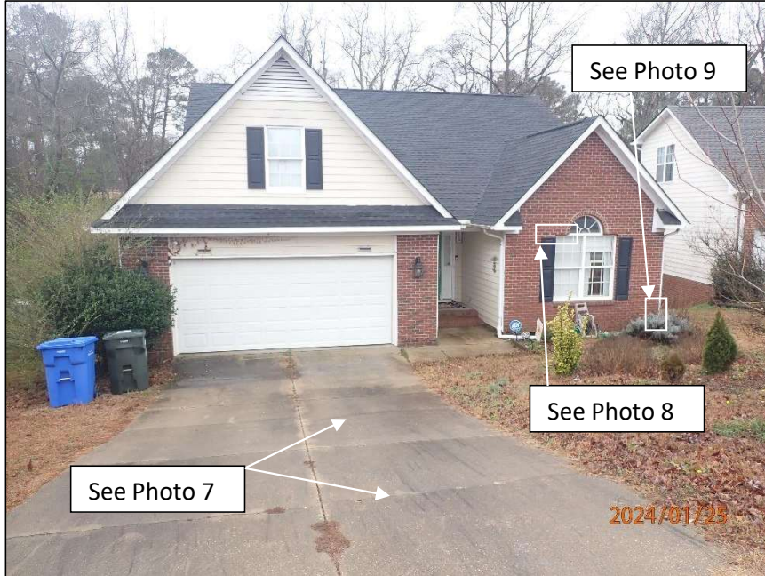
Photo 1 Area of residence observed – front elevation
