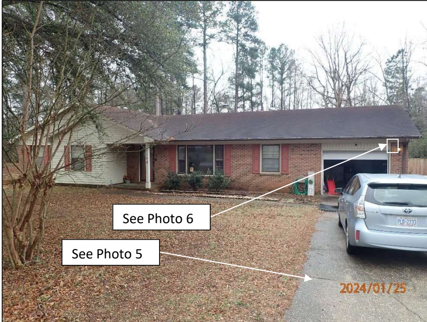
Photo 1 Area of residence observed – front elevation
