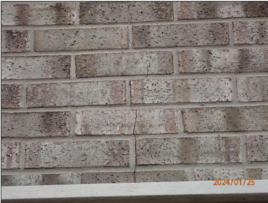
Photo 6 Vertical crack
