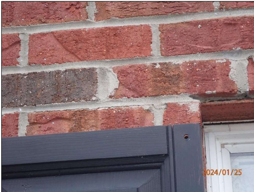
Photo 8 Horizontal crack
