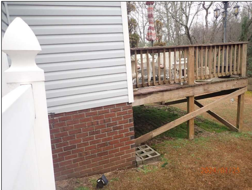
Photo 4 Area of residence observed – back corner – backyard inaccessible
