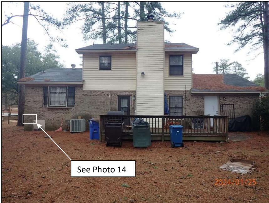
Photo 4 Area of residence observed – back elevation
