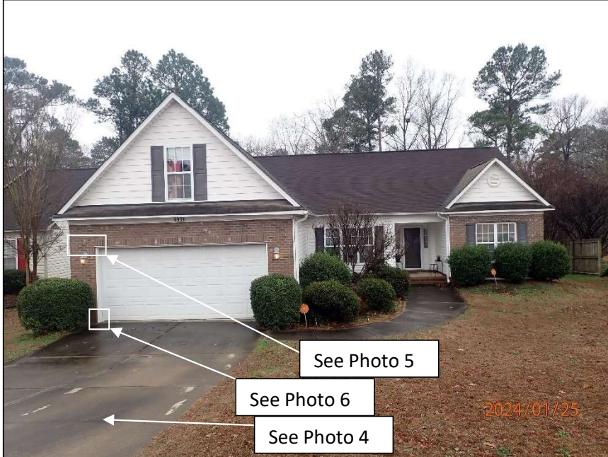
Photo 1 Area of residence observed – front elevation
