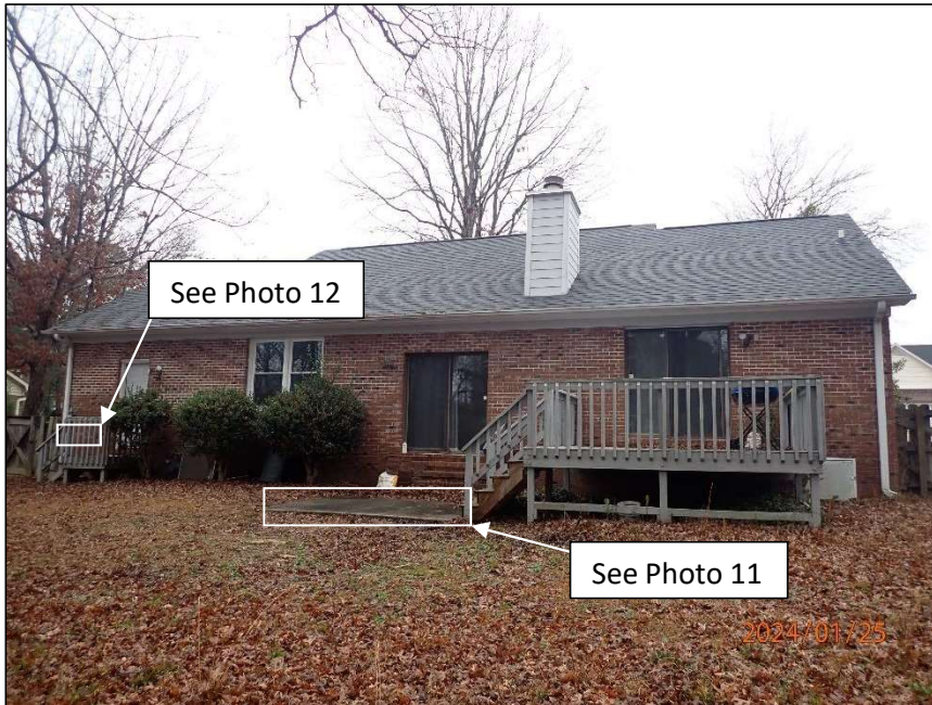
Photo 4 Area of residence observed – back elevation
