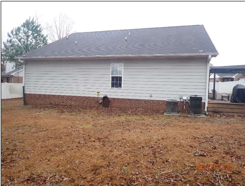
Photo 6 Area of residence observed – back elevation
