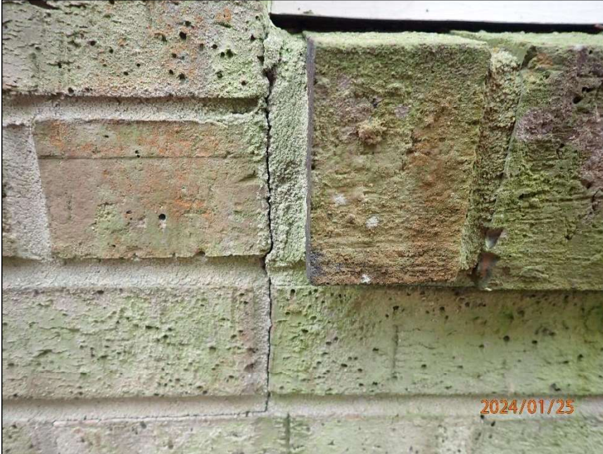
Photo 13 Step crack
