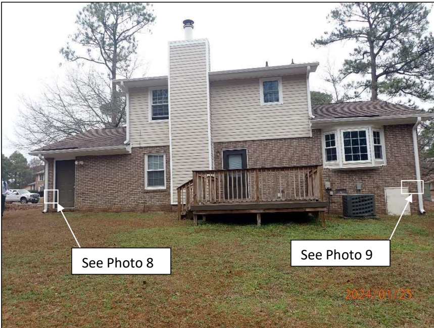
Photo 4 Area of residence observed – back elevation
