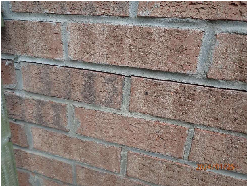
Photo 8 Horizontal crack
