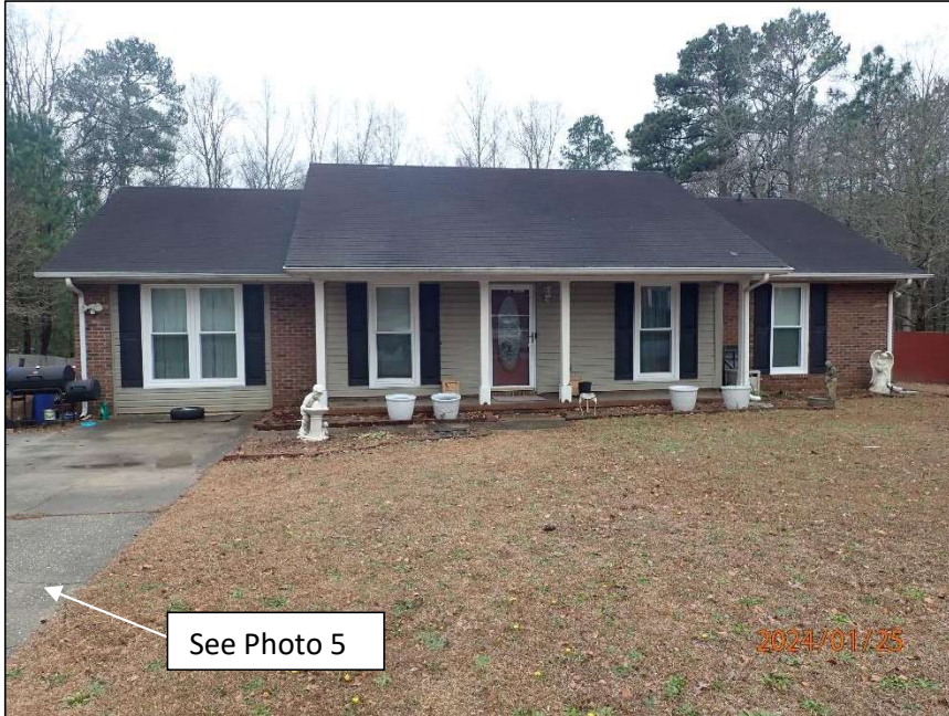
Photo 1 Area of residence observed – front elevation
