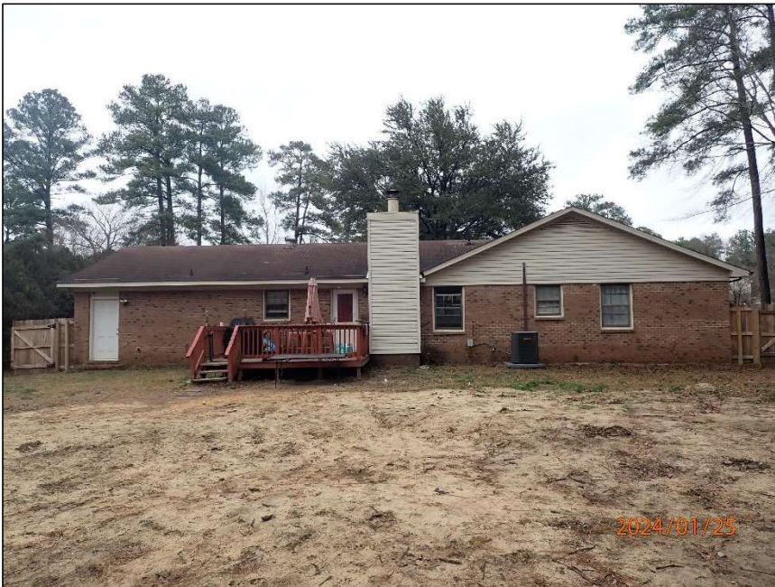
Photo 4 Area of residence observed – back elevation
