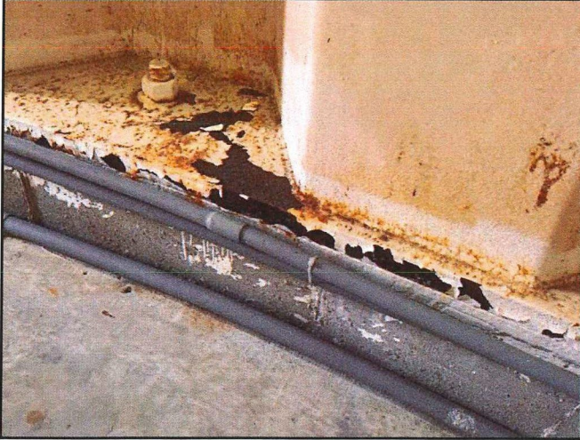
Photo 11 Corrosion at baseplate.
