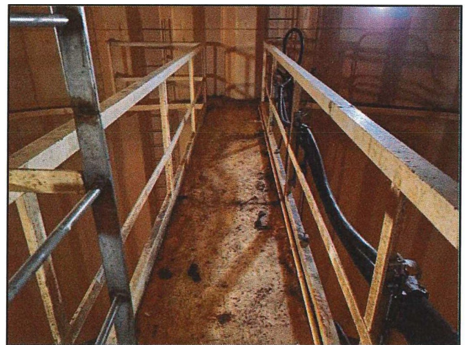
Photo 10 Manway below dry riser tube.
