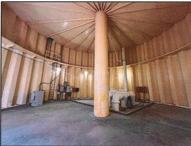
Photo 9 Interior dry below condensation ceiling
