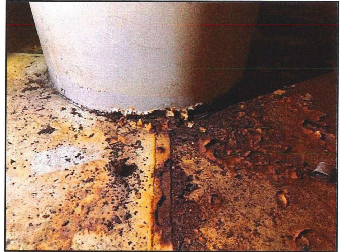
Photos Zoomed in at condensation ceiling interface with dry riser.
