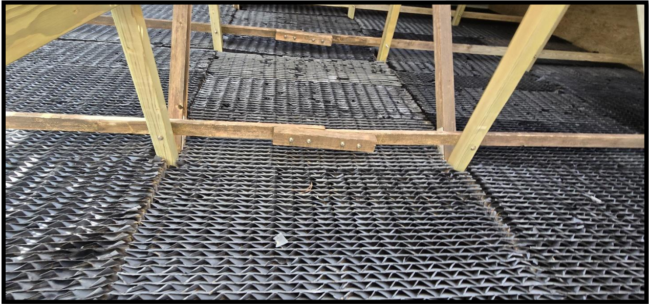
Typical material condition of the drift eliminator panels in all cells (bottom of page 3 and above).
