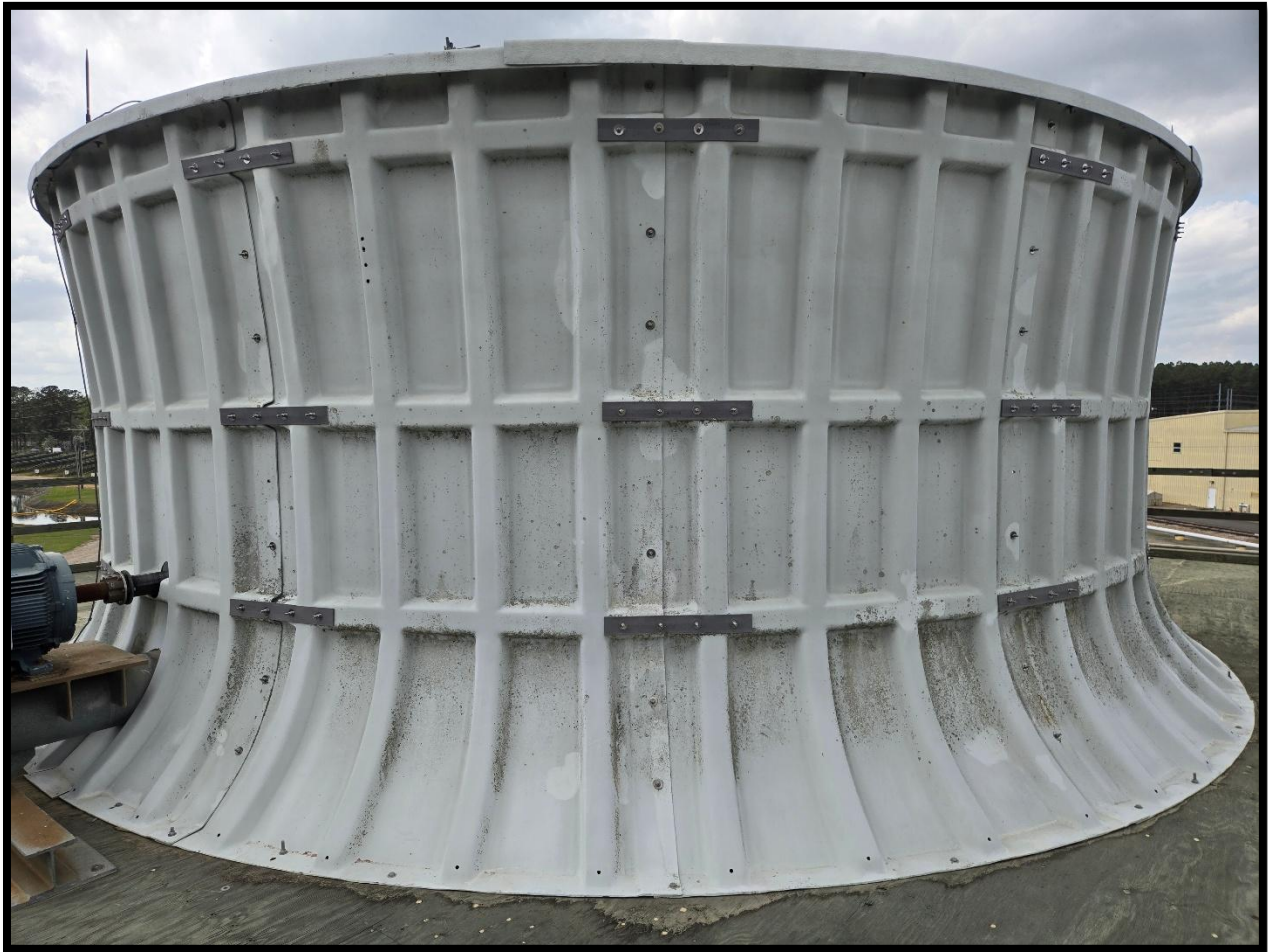
Typical material condition of the fan cylinders on all cells.
