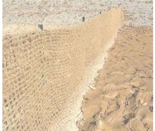
Figure 6.65d Close-up of a porous baffle.
