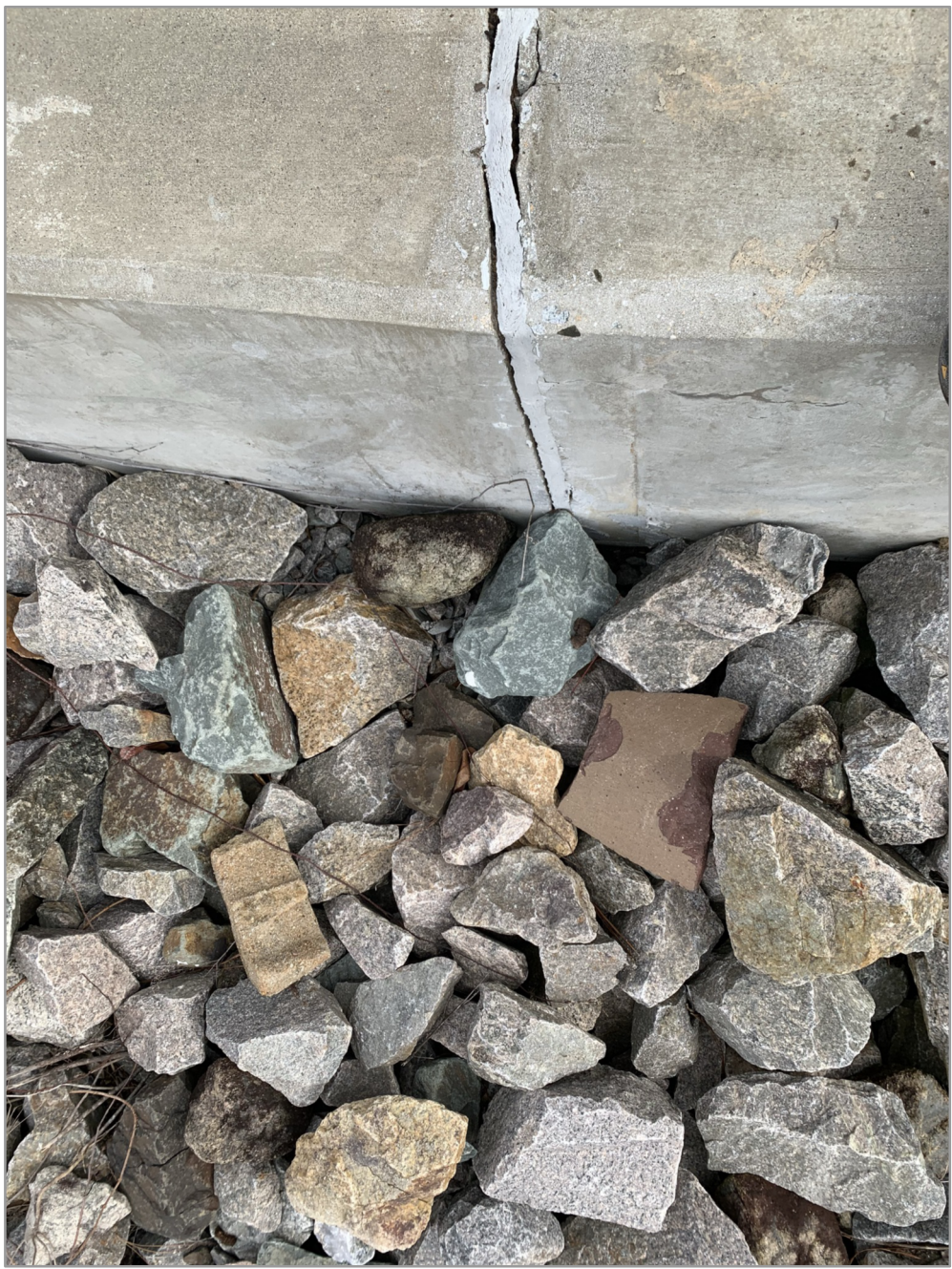
JOINT SEALANT REPLACEMENT (REFERENCE DETAIL A/S–2)
