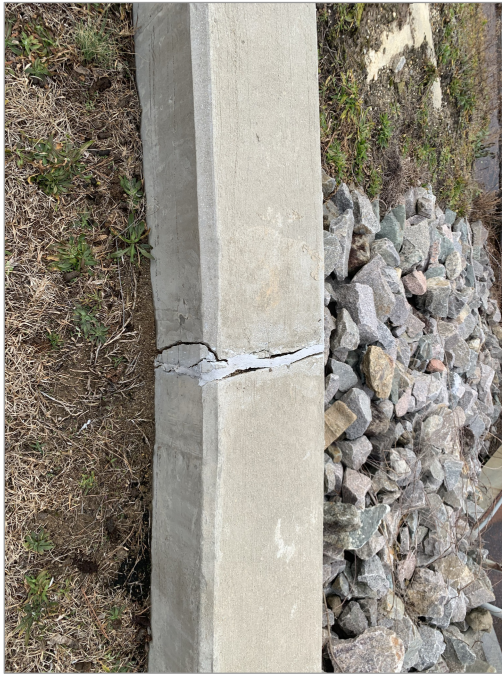
SPALL REPAIR/JOINT SEALANT REPLACEMENT (REFERENCE DETAIL B/S–2)
