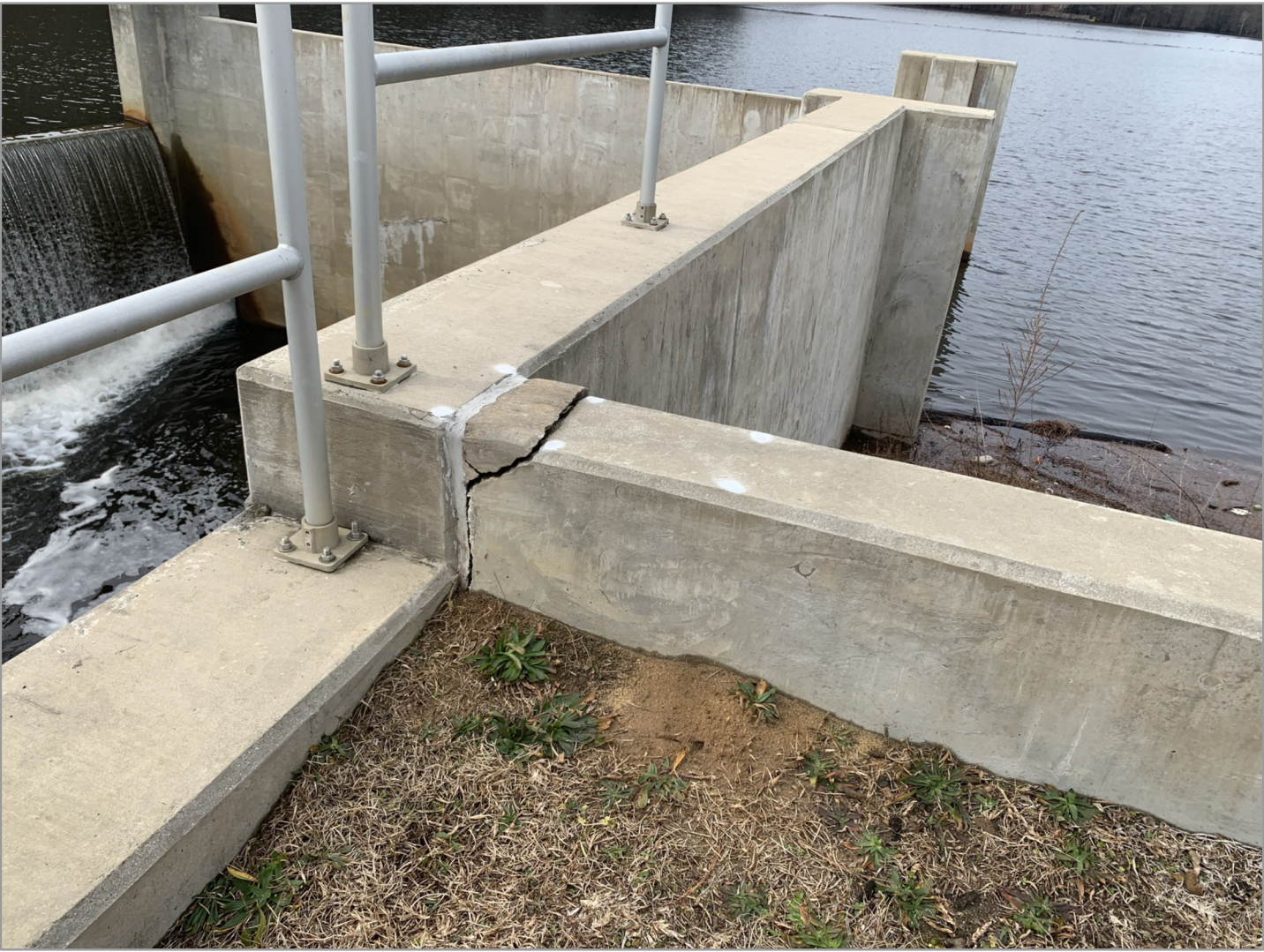
JOINT SEALANT REPLACEMENT (REFERENCE SECTION 1/S–2)
